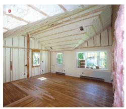
After cleaning up the demo mess, I called in my framing contractor and devised a solution. Building a second "roof" as we had originally planned would interfere with the new valley, so instead we decided to replace the existing ridge board with a ridge beam and let the underside of the rafters become our vaulted ceiling.
