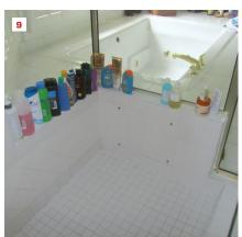
on site, and our subcontractors know to bring preformed outside corners and the correct adhesive for the material. We cover the curb completely, all the way to the floor.
