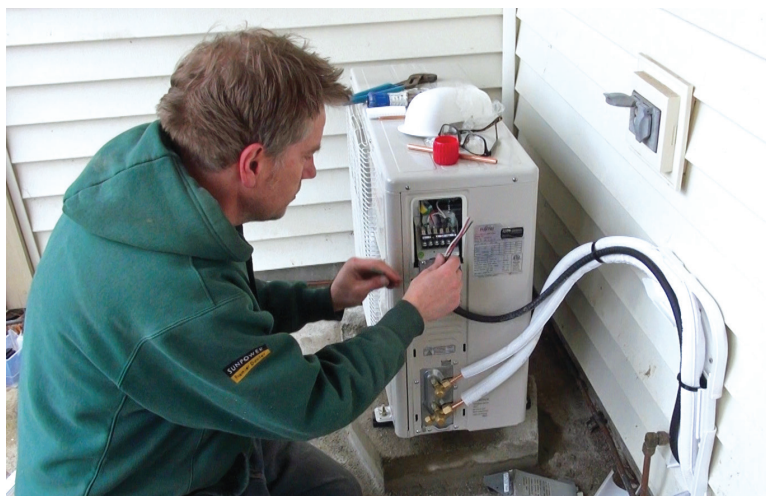
ReVision Energy's Dave Ragsdale connects the control circuit of the outdoor unit of a 1-ton Fujitsu mini-split on a home near Portland, Maine. In combination with a wood stove, the mini-split will mostly idle the home's existing oil boiler, except during the coldest part of the year.
