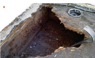
surfaces. This reaction happens even more quickly in salt air. The patina eventually creeps under the polymer waterproofing and causes it to debond.
