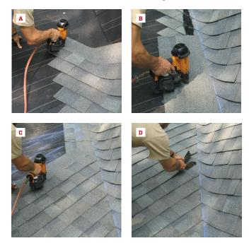
In the "Tamko" valley, one slope (the shallower, if applicable) is completed first, with its courses running through the valley by at least 12 inches (A). Next, full shingles are nailed end-to-end along a chalk line; a bead of roofing mastic adds insurance against uplift (B). The opposite slope is completed with square-cut corners toeing the valley line (C). A dab of mastic glues the sawtooth tips to the valley starter (D).
