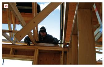
The following day we nailed off the ripped sheathing and shingled the eaves. It took about 12 man-hours total for two men working together to flash the smaller roof to the gable end of the larger roof section, despite the 20°F temperature.
