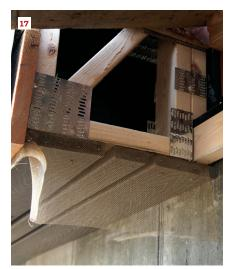
into magnesium-oxide board, which has a high perm rating, but transporting it to the island was prohibitively expensive. Instead, Baczek suggested that we sheath the trusses with rough-sawn pine boards (14), which were affordable, locally available, and vapor open. It was a perfect solution.
