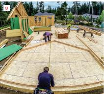
10. Now we can lay out the studs along the rake wall. Pulling from the left, the first stud is 16% inches to the long side of the stud. Again, using the Construction Master calculator, we calculate the distance along the top plate, this time using 16% inches as the RUN.
