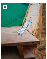
the overhangs to fit LP SmartSide Soffit, which comes in 12-, 16- and 24-inch-wide panels. To accommodate expansion, we frame the overhang ¼ inch wider than the soffit material.
