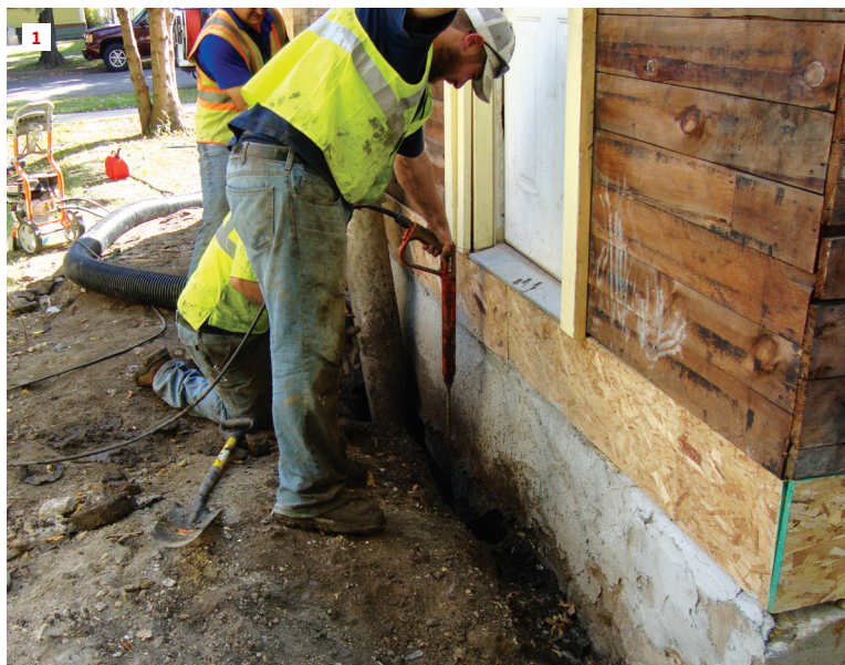
A "water knife" (a power washer) is used to slice a narrow slot around the perimeter of a house in Minneapolis. The Building America project successfully demonstrated that exterior foundation insulation can be cost-effectively retrofitted on existing homes to boost energy savings and help control moisture migration through the foundation.
