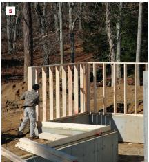
one stud length. Fortunately, we were working behind a good form contractor on this job and were able to work within our ½-inch tolerance. If the foundation hadn't been level, we would have adjusted the stud lengths as necessary to ensure a level first floor.
