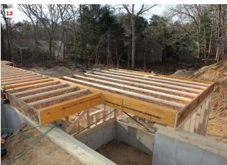
full-height foundation walls. Then we run a second KD sill plate around the perimeter of the foundation (8) that laps onto the drop walls as the second top plate. Again, we make sure that we lap all seams and corners. We also lap on to the framed drop walls wherever possible.
