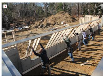
and attach a PT 2x8 nailer using 1%-inch powder-actuated fasteners. At the beam pocket, this nailer laps over the top of the mud sill, tying the beam to the exterior wall. At the other end of the beam, we let the nailer overhang by a couple feet to tie into the next section of beam.
