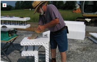
90°), brick ledges, and taper tops are available. Some manufacturers offer knocked-down components that are assembled on site: some offer both knock-down and fixed-dimension varieties. Most manufacturers' blocks are reversible top and bottom. For example, a corner block can be flipped over to create a left or right corner (1). Self-aligning nubs keep the blocks in place (2).
