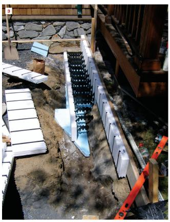
my favorite way to lower foundation costs. ICFs lend themselves to a variety of FPSF approaches. They can be used as concrete forms when shaping a turned-down (or "thickened-curb") concrete slab, or they can be stacked two (or more) courses high to create a crawlspace.
