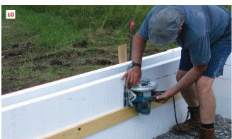
a full block on top—an overall height of 24 inches. We cut off the nubs on the outside edge of the top course (7) before capping it with 2½-inch lightweight channel to make screeding easier (8).
