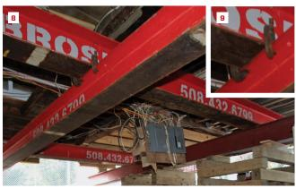
actually was because we had to set up temporary cribbing stations at various locations under the front part of the building to support it while we excavated access points for the main beams through the old foundation. Ultimately, each of the two main beams rested on four cribbing stacks, two inside the foundation at the front and two outside the foundation along the rear addition.
