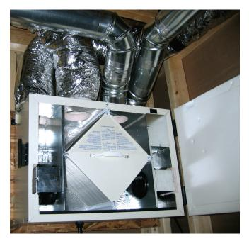
An HRV is just an insulated box with two fans, four ducts, and a recovery core (the diamond-shaped part in the middle). As the two airstreams go through the core, they exchange heat. They do not add heat to a house, but they will slow-down the loss of heat associated with providing fresh-air ventilation.
