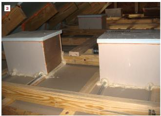
air-sealed exterior sheathing and airtight drywall on the same enclosure. Remember, we're talking about an air barrier, not a vapor retarder; there's no harm in having a double-sided air barrier. In fact, Energy Star requires that insulation be installed "in full contact" with *both* a sealed interior and an exterior air barrier.
