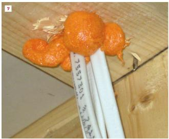
In an unconditioned attic, the sealing can be done from above any time before the insulation is installed (8).
