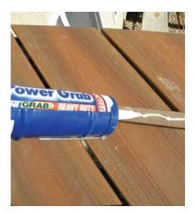
Loctite Power Grab adhesive is spread onto the back of the trim prior to installation. Power Grab dries clear, so if any squeeze-out is missed during cleanup, it's usually unnoticeable.
