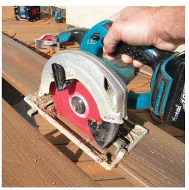
The trim can be cut on a table saw, but using a circular saw equipped with an edge guide is probably easier. The advantages to using a cordless circular saw are that it's lightweight and it has enough power for this cut. A 20-foot length of square-edged Fiberon Horizon decking yields 40 linear feet of 3%-inch-wide edge trim; the author sometimes uses a different width, depending on the brand of decking he's working with.
