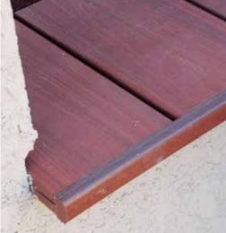
If you install capped composite decking, you know how unsightly the ends of the boards are compared with the capped tops, bottoms, and edges. One way to hide the ends is to install a border around the perimeter of the deck. While that can add visual interest to solid-color decking boards, it requires considerable blocking and adds to the project time line and overall cost. And when used with multichromatic decking boards, borders are almost a distraction.
