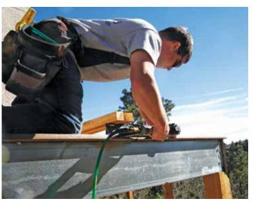
Eighteen-gauge stainless steel finish nails hold the trim in place until the glue dries. One nail per deck board is more than enough. ❖
