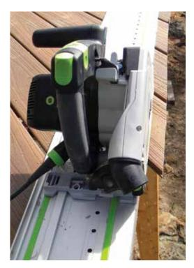
Deck boards are installed long and then cut in place along a straight line so the trim will lie flat once it's attached. A track saw, like the Festool TS55REQ shown above, is ideal for the job.
