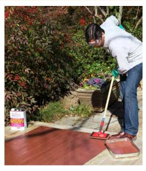
Repeated swelling and shrinking of a wood deck board can cause a finish to fail. Thompson's says its new WaterSeal Waterproofing Stain has a flexible film that can expand and contract with the wood, reducing cracking and peeling.
