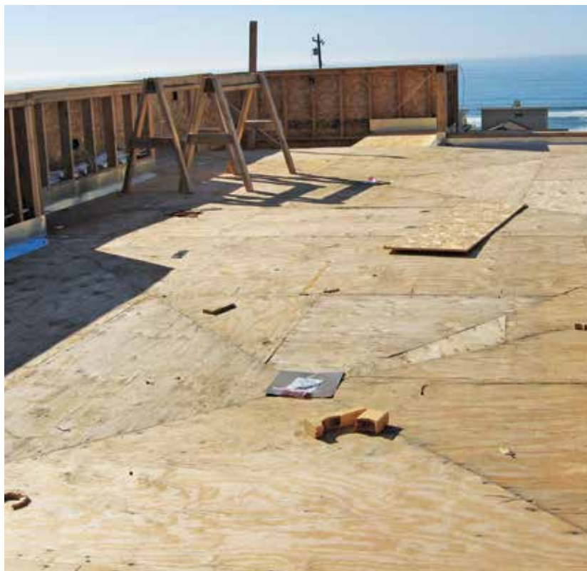
Figure 2. This large rooftop deck features two center drains, and was framed to slope the sheathing toward the drains. Most roof-covering manufacturers require plywood rather than OSB sheathing as a substrate.
