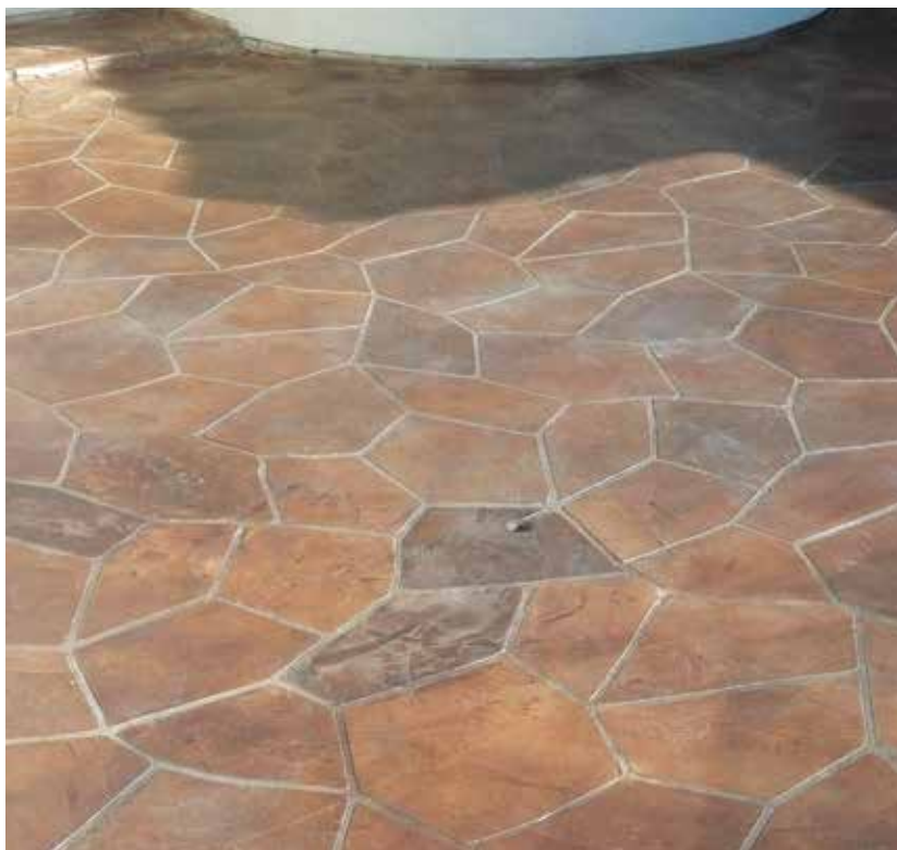
Figure 6. Cementitious coatings like Desert Crete are applied over metal lath stapled to the plywood sheathing. Chopped fiberglass mat is then glued to the base coat with acrylic resin, which acts as an anti-fracture and waterproofing membrane. After it dries, a protective screed coat is applied, with additional material helping to slope the surface for drainage, as required (top left). For a final finish, the deck can then be completed with tile or a spray-on textured finish (top right). Another option is to apply a stamped and stained finish to the deck, using heavy rubber templates laid into a wet skim coat of polymer concrete over the base coat to create the pattern (above).
