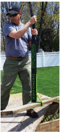
Once a board has been pulled from the joists, the tool can be used to quickly pick it up and move it out of the way.
