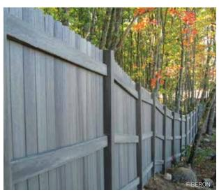
Routed (rather than bracketed) rail-to-post connections can be installed so that the fence follows the contour of the land.
