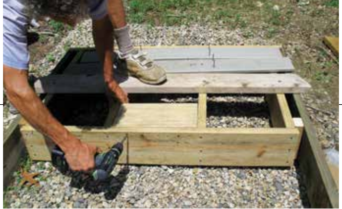
(A) Double blocking is stronger than single blocking, and screws hold better than nails. The author attached two blocks to the rim, joists, and vertical block (not yet installed) using four screws per block per side. Blocking installed parallel to the rim joist, as shown above, tended to split along the bolt line unless a heavy steel reinforcing plate was used.
