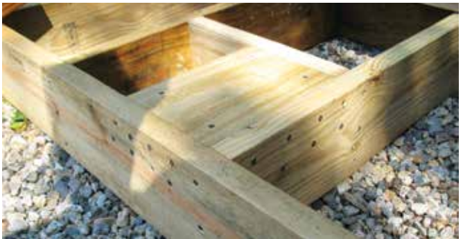
(B) The strongest blocking runs perpendicular to the rim joist. It's best to align the blocks with a nearby joist for extra stiffness and add a solid block between the rim and first inboard joist at the ends of the deck.
