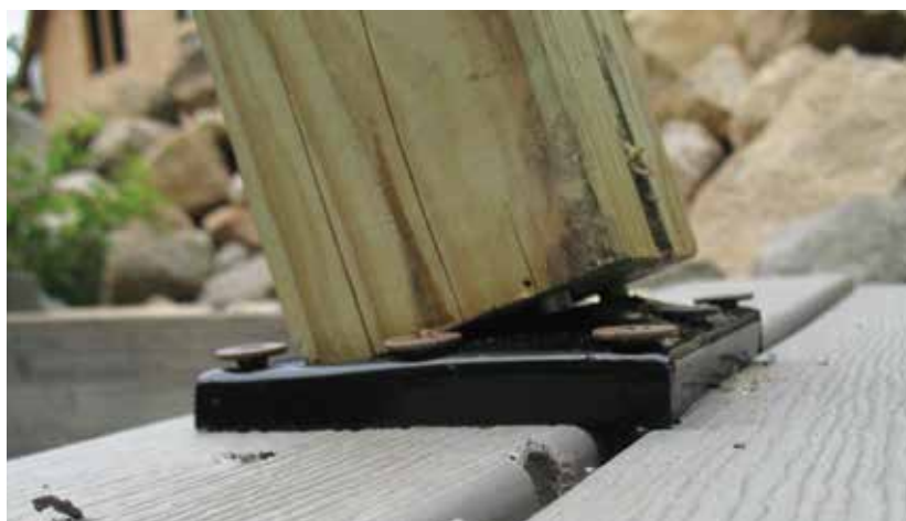
Figure 5. The Titan Post Anchor requires lag screws to secure the base plate to the post and 3-inch-long screws to fasten the base to the decking and blocking. Accessories such as a 1¼-inch-diameter hole saw (for drilling a mounting hole into the center of the post), a hammer cap, and a hole-saw centering tool are also available from Titan (above left). When the anchor was installed according to instructions, the inner screws pulled out of the blocking and decking at between 220 lb. and 270 lb. of force (above center). Using double blocking with the grain parallel to the tension force and through-bolts and washers instead of screws improved performance, but the top of the post deflected almost 12 inches (above right) before the bottom of the post finally split at 374 lb. of tension (right).
