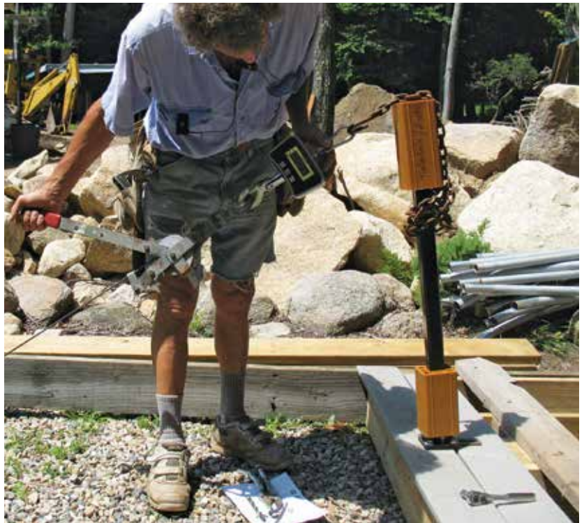
Figure 2. The TimberTech/Azek post is sold separately from the install kit, which includes an adjusting plate and adjusting screws along with a reinforcing bottom plate and bolts (top left). The top block has set-screw locations to lock onto the post for 36- and 42-inch-high railings. Anchor bolts drop through the holes at the corners of the base, while the smaller holes in the edges are threaded for the adjusting screws that are used to plumb the post (bottom left). The 3½-inch-square bottom of the post shows no signs of bending after testing at 500+ lb. of tension (above).
