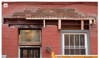
reached the outer channel, he punched in from the outside. Then he used 1/2-inch through-bolts to fasten the steel and wood together at both ends and in every third hole in between; he finished the bolting after the brickwork was completed.
