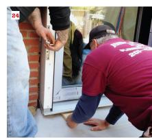
be installed first and panels set in place, we thought it would be easier to put the heavy panels together working flat on the deck. At about 9 feet square and 900 pounds, the door was still within the limits of what we believed we could lift into place.
