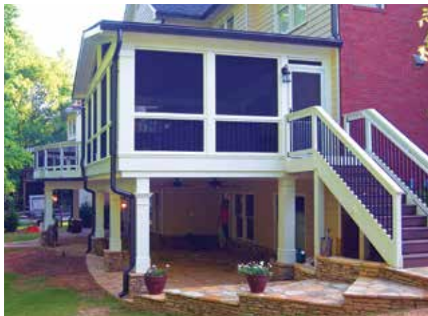
Figure 6. The author prefers to set flagstone patios and walkways in mortar over a concrete slab rather than over a sand or crushed-stone base. This method requires more attention to drainage details, because water can't seep through the joints between the stones.
