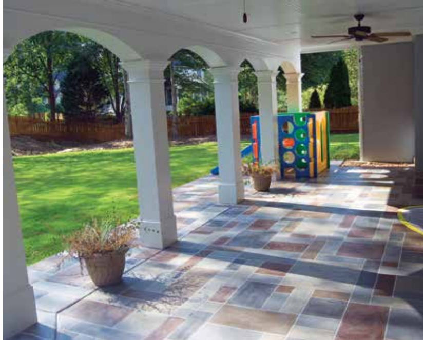
Figure 3. When a concrete slab has been extended, a thin concrete coating can be used to visually tie the old and new slabs together. The coating shown here has been stamped and colored to look like natural stone.
