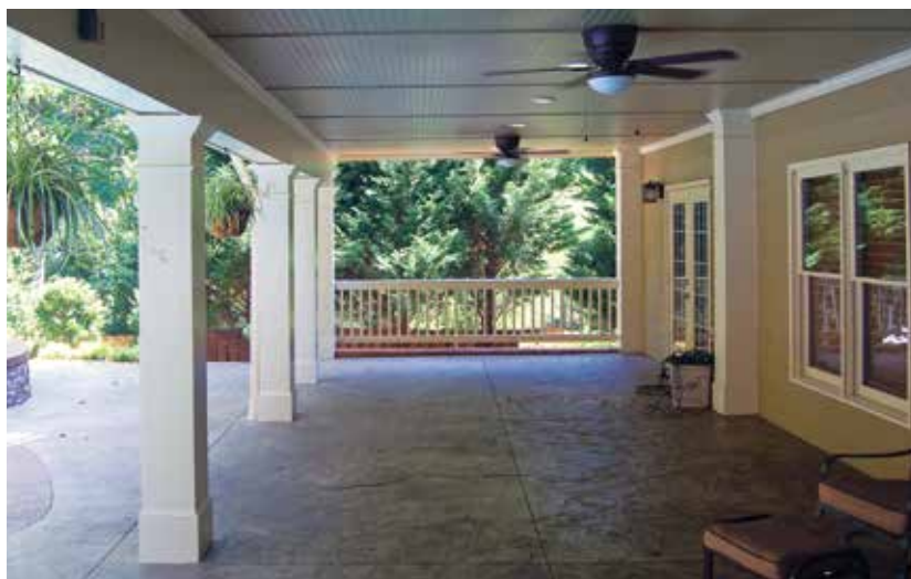
Figure 4. The flat, smooth finish of stamped concrete makes it well-suited for a screened-porch floor. Note the expansion joints, which are more noticeable in the faux flagstone floor (above, left) than in the larger random pattern at left, where the relief joints make the patio appear to be composed of large slabs of slate.
