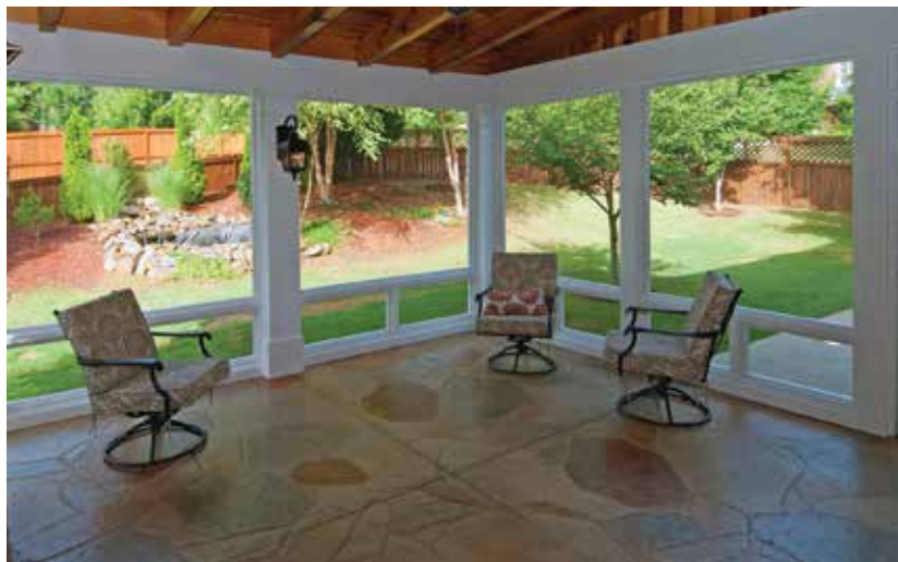
Figure 3. When a concrete slab has been extended, a thin concrete coating can be used to visually tie the old and new slabs together. The coating shown here has been stamped and colored to look like natural stone.
