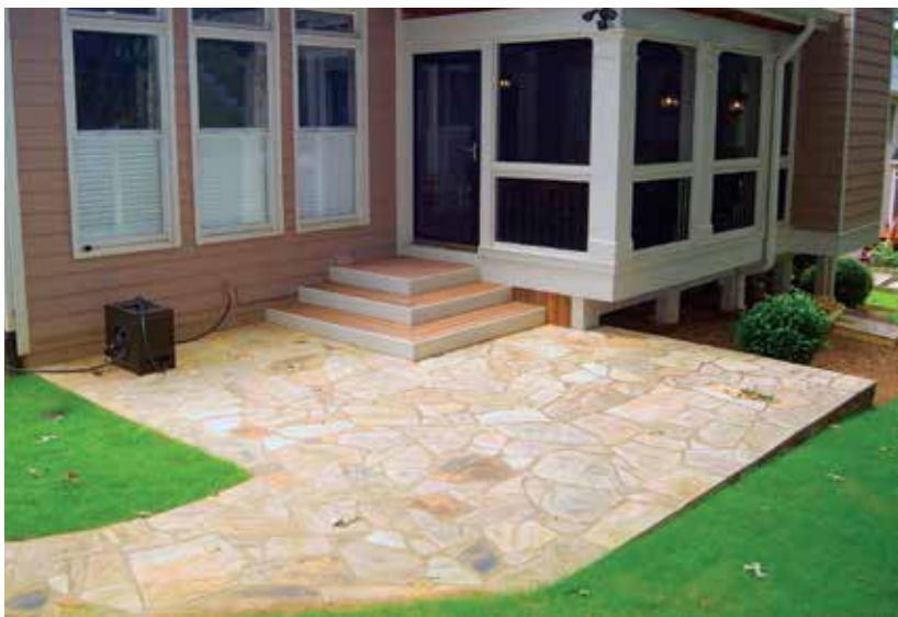
Figure 1. On a level site where the interior floor is close to grade, a patio is often a better and less-costly option than a low-elevation deck.
