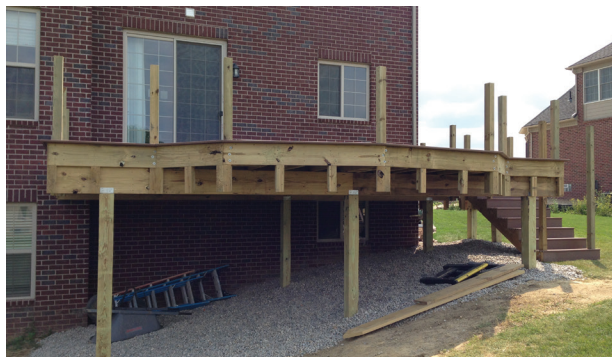
Drop blocks were added to the cantilevered section of this deck to support tiered trim that will be used to finish the fascia.
