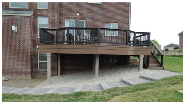
With finished support columns and tiered fascia, this raised deck looks good from the ground level.
