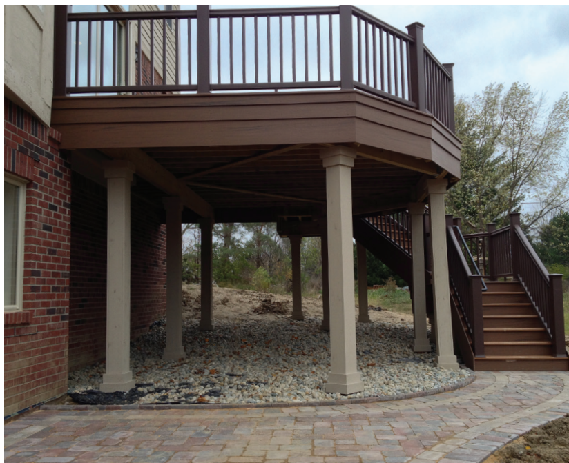
Clad support columns that have been stained to match the trim on the rest of the house look more substantial than bare 6x6 PT posts and do a better job of visually anchoring a tall deck to the ground.
