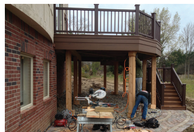
Offcuts were used for the simple built-up trim applied to the bases and tops of the cedar-clad columns.
