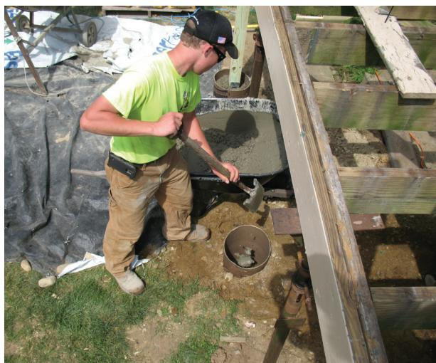
**Prescriptive foundation sizing guidelines are based on bearing area and don't account for the weight of the concrete used to form deep footings and piers.**
