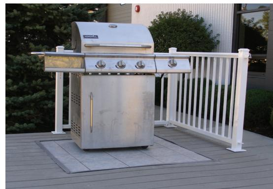
Deck joists should be placed 16" O.C. TI-ProBoard® comes in 12" widths by 8' or 12' lengths For more information visit our website.
