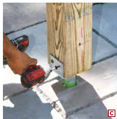
Figure 2. Instead of concrete tube forms, the author uses helical screw piers from TechnoMetal Post (A), which can be installed with a small gas-powered machine and barely disturb the landscape. The piers are capped with a metal post bracket (B); four HeadLok screws secure the post (C).
