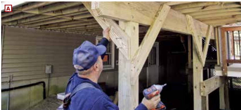
Figure 3. The author's crew installs Y-bracing (A) to resist side-to-side movement parallel to the house. Lateral braces resist movement away from the house; these are installed from each post to the side of a joist (B) or to a block between joists (C).
