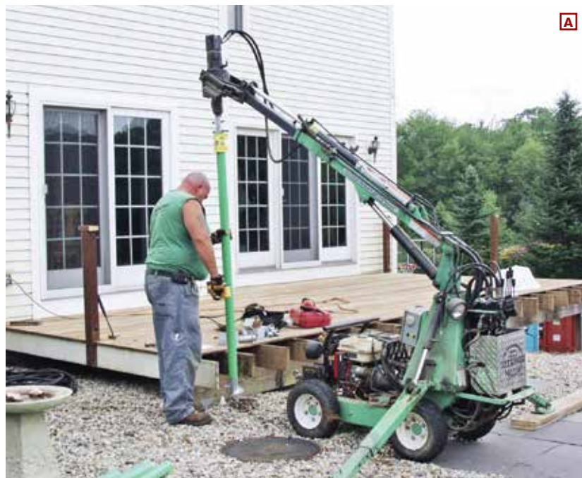
Figure 2. Instead of concrete tube forms, the author uses helical screw piers from TechnoMetal Post (A), which can be installed with a small gas-powered machine and barely disturb the landscape. The piers are capped with a metal post bracket (B); four HeadLok screws secure the post (C).
