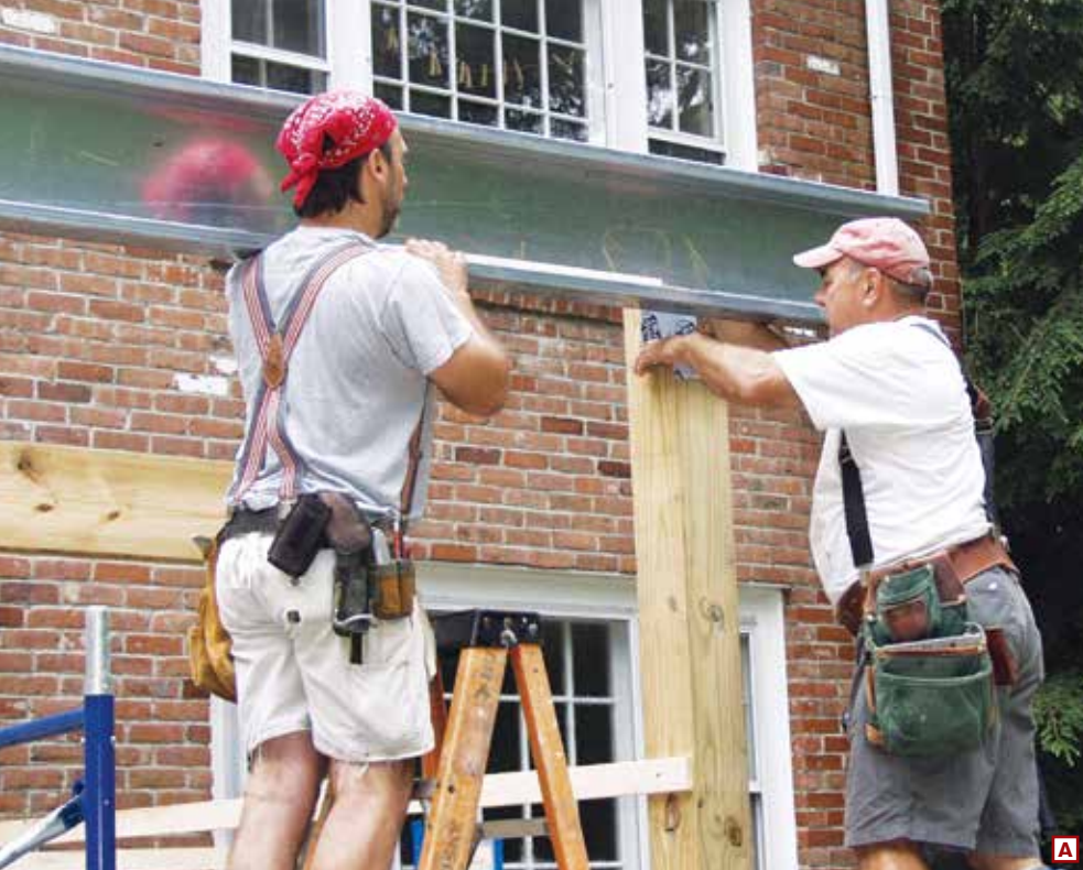
Figure 6. Using a LiteSteel beam enabled the author to eliminate a view-obstructing post in this deck project (A). Two-by-squash blocks (B), secured with ThruLok bolts (C), cinched the connection to the notched post.
