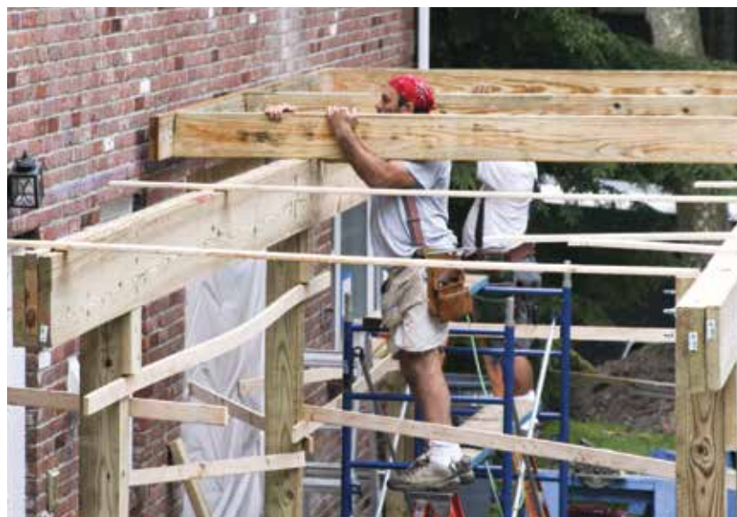
Figure 7. Carpenters set the joists for the freestanding deck; the band will remain spaced away from the brick veneer wall. Where joists cross the LiteSteel beam, strips of flashing membrane separate the pressure-treated lumber from the steel.
