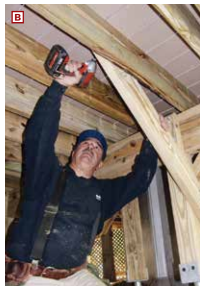
Figure 3. The author's crew installs Y-bracing (A) to resist side-to-side movement parallel to the house. Lateral braces resist movement away from the house; these are installed from each post to the side of a joist (B) or to a block between joists (C).
