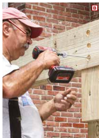
Figure 1. ThruLok screw bolts (A) provide a quick way to assemble built-up girders. They self-tap, like many wood screws (B), and are secured on the back with a wing nut (C).
