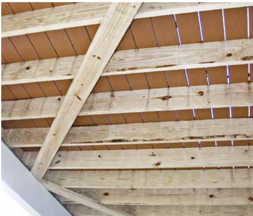
Figure 4. Whenever the decking is installed perpendicular to the joists instead of diagonally, the author uses 2x6 V-bracing to resist racking. The V-braces are attached to each joist with two screws. V-bracing is also used with many brands of grooved composite decking, which is typically installed with clips that do not resist horizontal forces.
