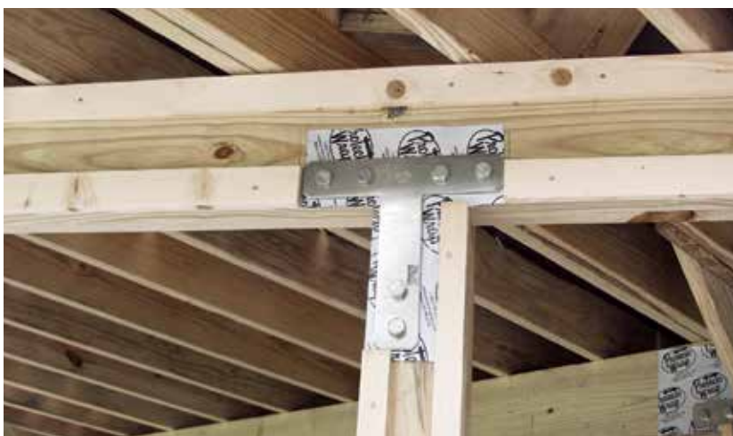
Figure 5. In cases where Y-bracing will obstruct views from doors or windows under the deck, the author substitutes rated metal T-straps at column-to-beam connections.
