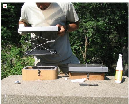
finish dimensions of flue liners, the damper frames have wide flanges and may hang slightly inside or outside the flue liner opening.
