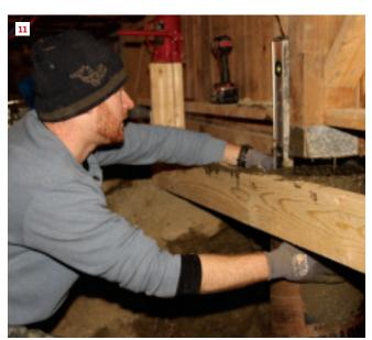
the piers out by hand, one at a time. That crew also set disc-shaped precast concrete footings in place, 6 inches thick by 24 inches in diameter.
