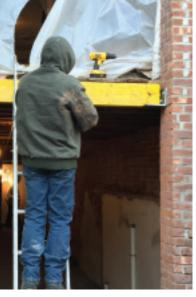
match the existing joist depth (12). We weren't too concerned about compromising their structural integrity; in this case, the LVL was essentially just blocking. However, the clients are thinking about adding a deck off the kitchen in a year or so, and the LVL should provide good anchoring for a ledger, if they choose to do that.
