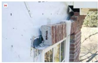
serve as a counterflashing to the stepped L-flashings that the roofers wove in with the new roof shingles.
