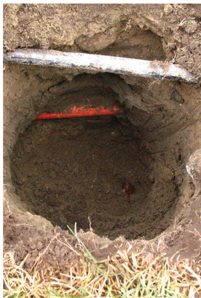
Figure 1. Before digging footing holes, call 811, your local utility locator. It will find and mark utility lines, but dig carefully; this service doesn't typically locate sprinkler lines, and here it missed a telecom cable conduit, too.
