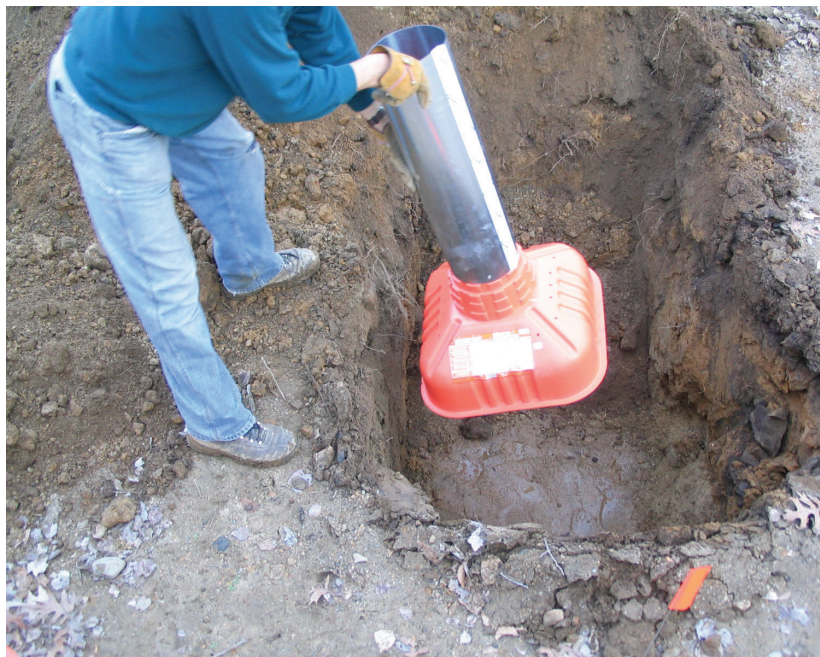
Figure 4. You can form piers using metal duct, which costs 30% to 40% more (about $4 more per footing) than cardboard tubes, but is more durable in wet conditions. To reduce costs, the author recycles his HVAC sub's offcuts, as well as old ductwork removed from remodeling jobs.
