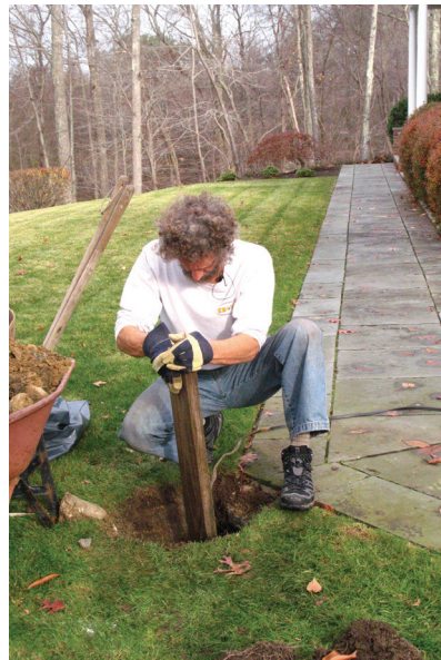
Figure 3. Alternatively, loose soil can be compacted with a tamper, a framing offcut, or with a section of a 4x4 or 6x6 post.
