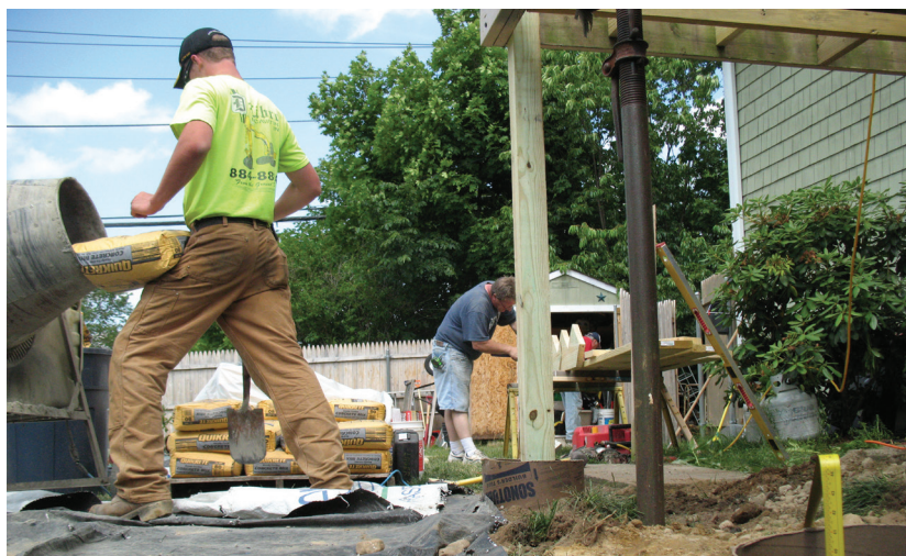
Figure 7. A pier should extend a few inches above grade so that the hardware used to connect the PT post to the pier won't get covered with soil.
