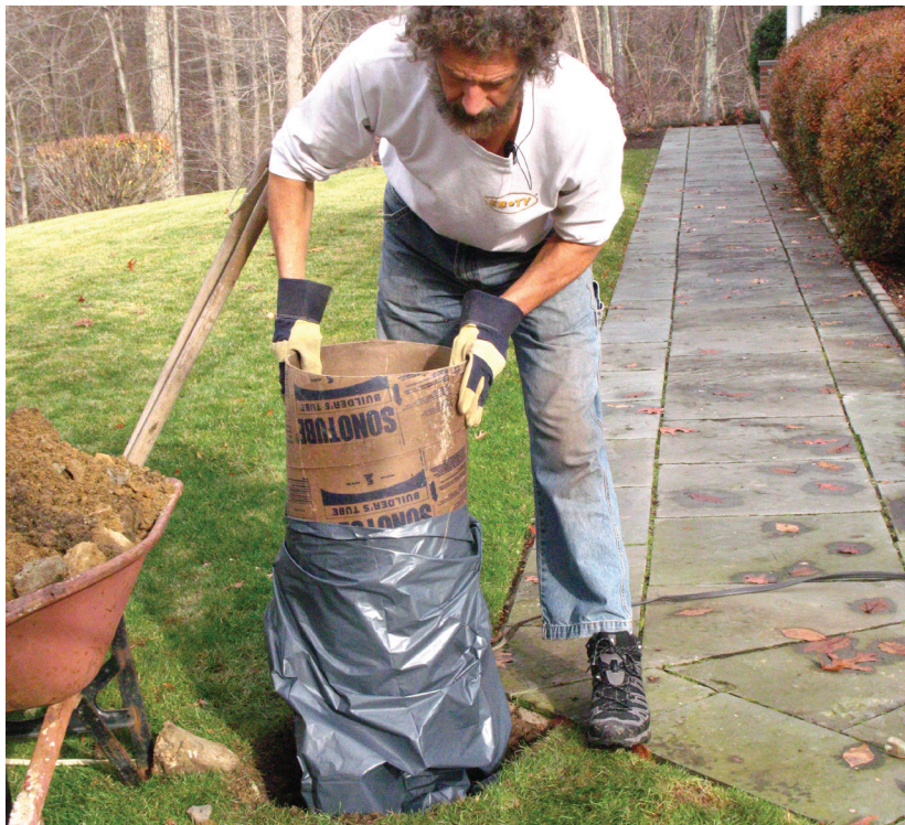
Figure 6. Garbage-bag footing bases are useful in wet conditions, as well as when your footings will be wider than concrete tubes but smaller than prefabricated wide-base forms. The author digs a 12-inch-diameter footing hole about two-thirds of the footing depth, then widens the last third of the hole to the calculated size. After duct-taping a heavy-duty garbage bag to a footing tube cut 6 inches longer than two-thirds of the depth, he pokes rebar horizontally through the form 6 inches from the top to suspend the form in the hole. Finally, he pours concrete in the bottom third—the bag—then backfills the space between the hole and the form before filling the form to the top with concrete.
