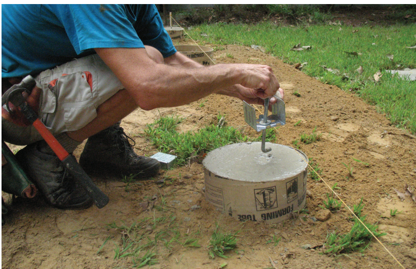
Figure 9. After the author pours concrete into the form, he makes sure the top of the pier is flat, rather than angled or crowned. Sloped tops make it hard to set a post base properly.
