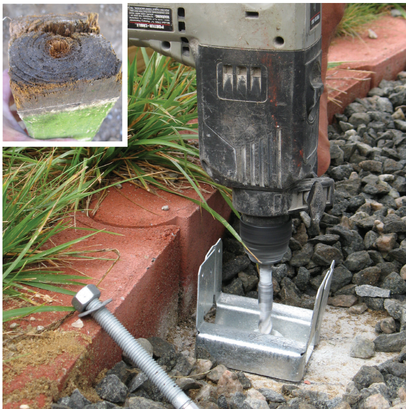
Figure 8. Most post bases have an elevated plate that prevents the bottom of the 4x4 or 6x6 post from coming in direct contact with the concrete. Even though PT posts are treated for ground-contact, end grain will wick up moisture and is particularly vulnerable to rot (inset).
