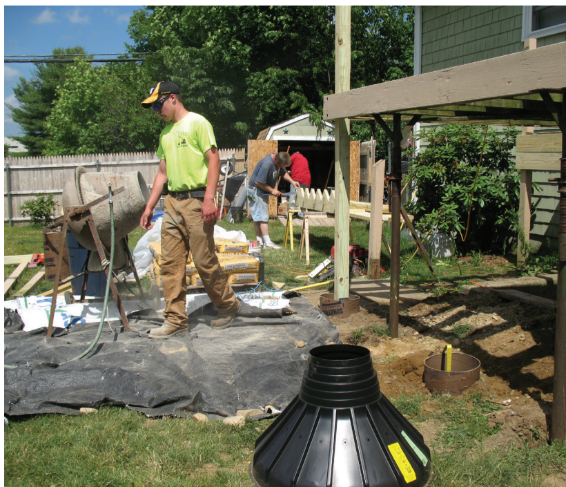
Figure 5. To increase a pier's bearing area without adding a lot to the total volume—and weight—of concrete needed to build it, many deck builders add a wide-base form to their standard cardboard-tube footing forms.
