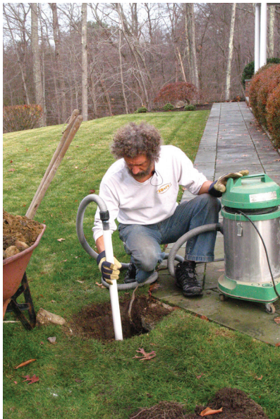
Figure 2. You're always disturbing the soil at the bottom of the hole as you dig and it's hard to scrape it out, especially from deep holes. One trick for removing the loosened soil is to vacuum it out.
