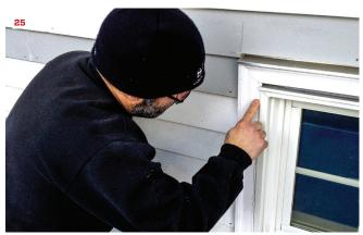
wood with quick-drying primer. Raw wood, like the cut ends of clap-boards, is vulnerable to absorbing moisture, which can cause paint to fail prematurely (or worse, can lead to rot).
