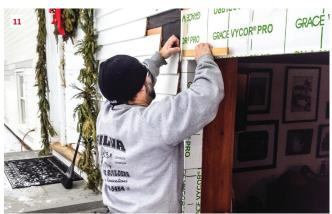
Cutting and installing these fillers took about a half-hour per window. The cost of my time and the few materials for the fillers worked out to be a lot cheaper than what the upcharge would have been for ordering custom-size windows to fit the original rough openings.
