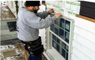
along both sides. Before I applied the flashing, I scribed a pencil line along the top and sides of the window about ¾ inch from the flange, using my finger as a guide. This line helped me place the flashing tape during the installation, and having the tape lap slightly onto the side of the window provided a better seal along the edges of the window frame to prevent moisture from entering.
