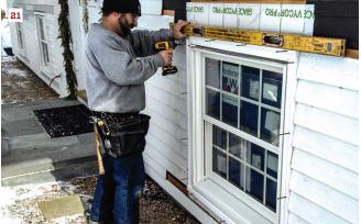
to know the angle of the sill where the sides would attach. To copy the angle, I laid the sill on its back and placed a scrap piece of casing against it. I traced the angle and then took the scrap to my miter saw and lined it up with the blade to set the angle of the cut.
