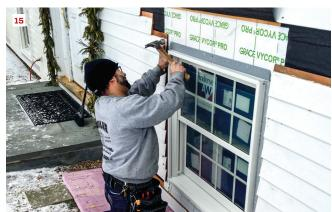
jamb until I reached the inner corner, using my layout square to press the flashing tight to the corner. I smoothed the outer face with my hand and again slid the flashing behind the siding and pressed it into place with a shim shingle (10).
