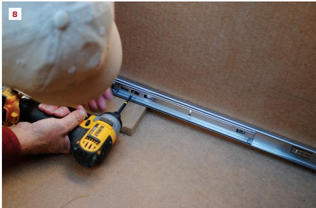
**5.** Cabinet bottoms were nailed in place, then more securely fastened with pocket screws.
