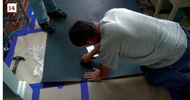
the viscoelastic adhesive absorbs even more sound energy and decouples the two layers of drywall from each other.
