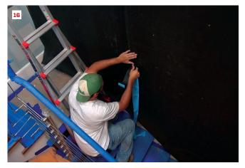
We replaced the foam insulation with special acoustic rock wool fiber batts. (We don't have an official sound-abatement contribution for either open-cell or closed-cell plastic foam insulation, but experience tells us that the relatively dense foam increases sound transmission through walls.)
