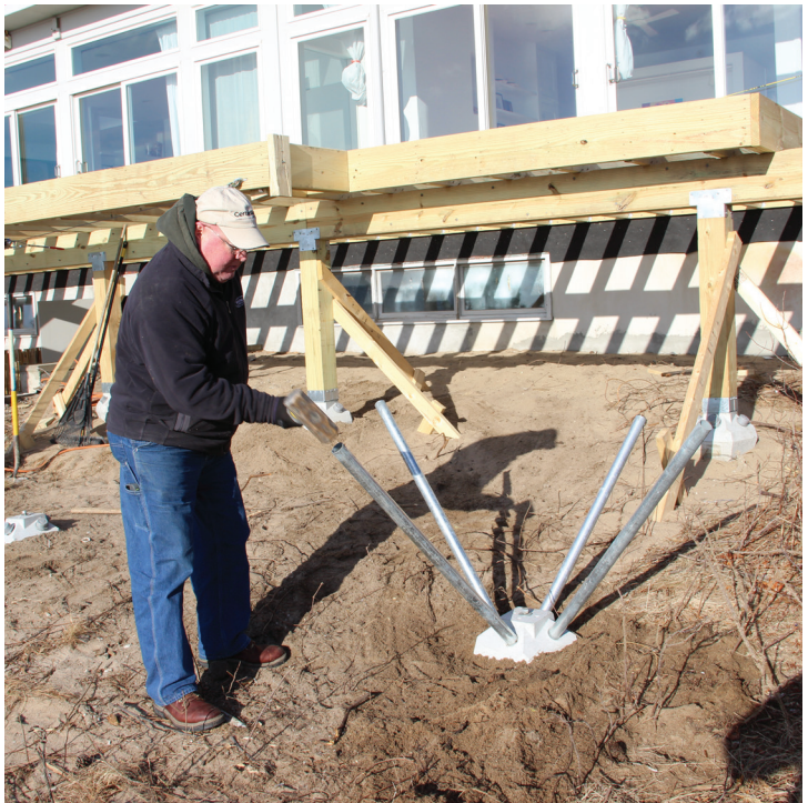
Figure 6. A sledgehammer is used to start the pins. In fact, it's possible to fully drive the pins with the sledgehammer in this relatively soft sandy soil.
