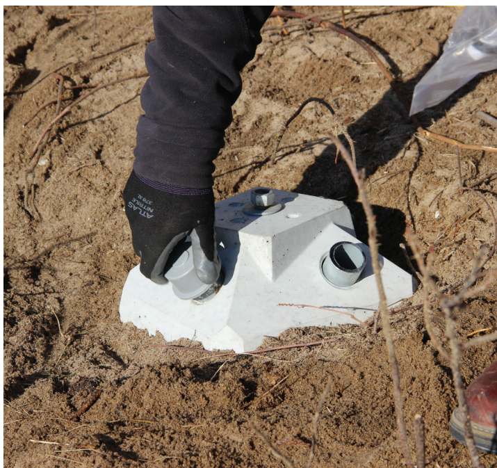
Figure 10. The pins are covered with plastic inspection plugs. They can be removed, allowing a building inspector to measure the pin's insertion depth with a tape and verify that the installation conforms to the manufacturer's instructions.
