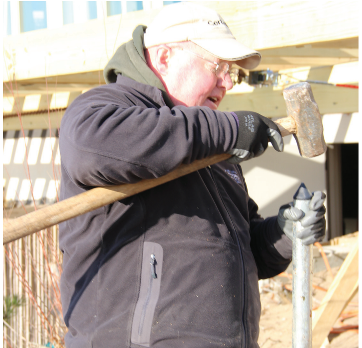
Figure 5. The pin piers come with plastic end caps that help the pin penetrate soil without filling up with dirt.
