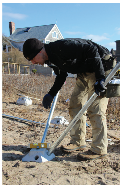
Figure 4. Fine adjustments can be made to the pier's position after the 2-inch-diameter galvanized-steel pin pipes are inserted into the guide holes in the pier head.
