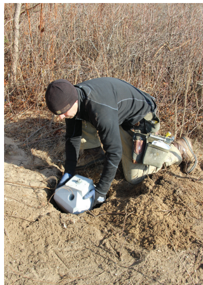
Figure 2. The pier heads come in various sizes. The DP75 piers used on this project weigh about 75 pounds each and can easily be handled by one man.
