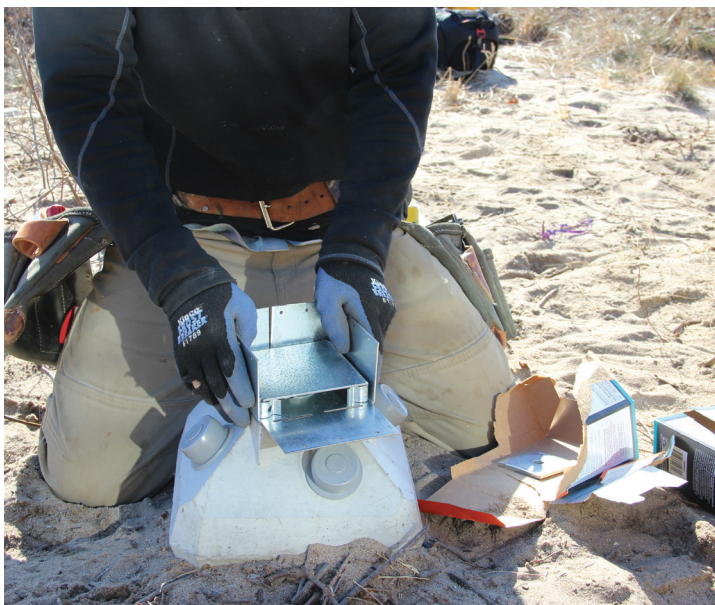
Figure 12. Given suitable soils, a single worker can set all the piers for a typical residential deck in an hour or two and be ready to start framing.
