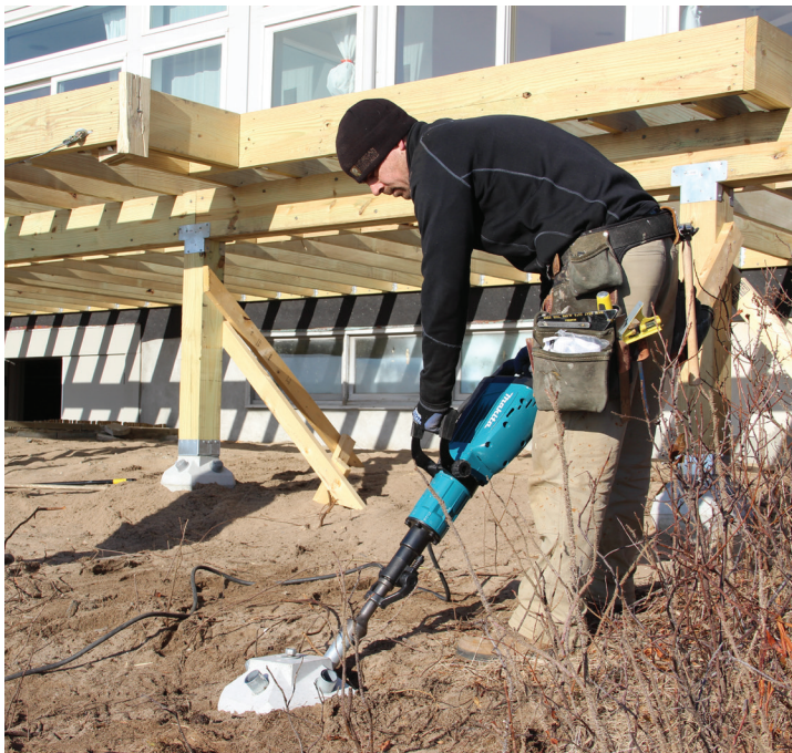
Figure 9. When a pin is fully set, the driver bit bottoms out on the pier, leaving the head of the pin standing about 1½ inches proud of the pier.
