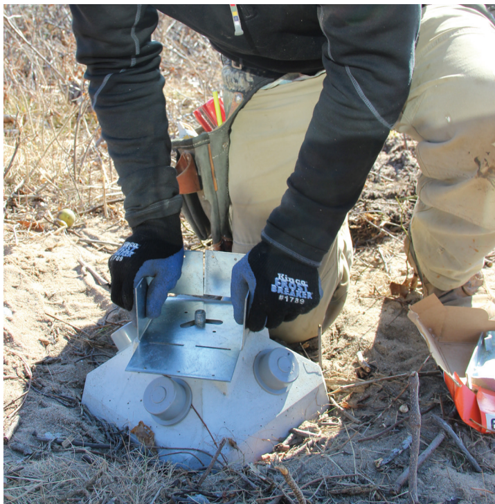
Figure 11. Once the pier head is pinned to the soil, a post base or other metal hardware is fastened to the pre-installed bolt embedded in the concrete.
