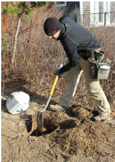
Figure 1. A Diamond Pier footing head can be placed in a shallow hole, because deck loads aren't actually supported by the soil beneath it. Instead, loads are transferred to the soil by pins driven through the pier.
