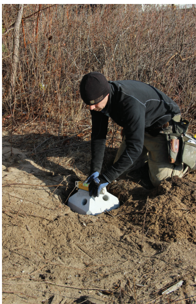
Figure 3. After a quick check with a torpedo level, the pier head is ready to be pinned to the soil.
