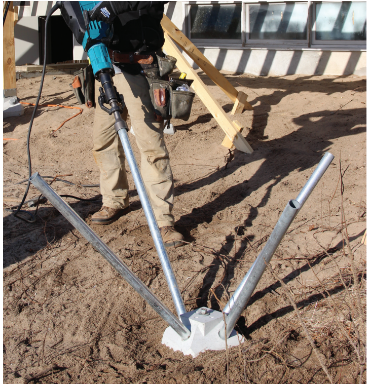
Figure 7. With a demolition hammer and special pin driving bit, it takes less than 10 minutes to fully drive all the pins for a pier.
