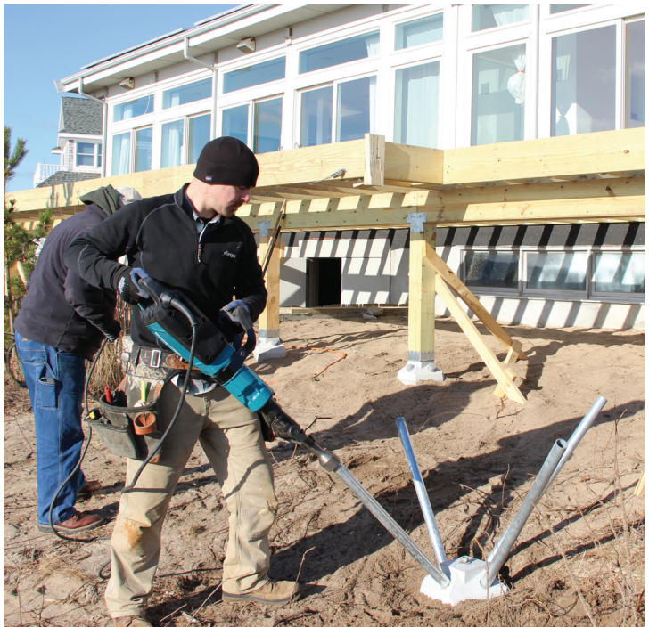
Figure 8. The installer works his way around the pier head, driving each pin about a foot at a time before moving on to the next pin.
