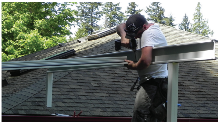
Figure 5. With the ridge I-beam in place, the T-bar rafters that will support the glazing panels can be screwed to the I-beam on 4-foot centers.
