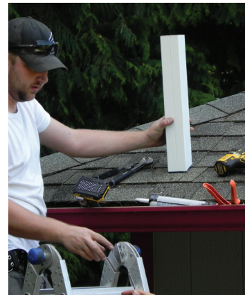
Figure 4. One end of the ridge beam supporting the patio cover's gable roof will be connected to this short post section, which fits over the post-bottom shoe.
