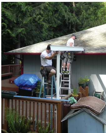
Figure 7. Because the cover section that will be supported by this beam will drain into a gutter, it has been slightly sloped back toward the house.
