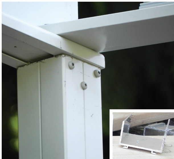
Figure 2. Beam-to-column connections are made by sliding post-top shoes (inset) into an I-beam's bottom channel, then inserting the shoes into the tops of the columns.
