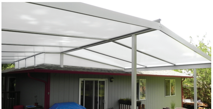
Figure 14. To keep water from splashing off the house roof and down onto the deck, this patio cover has optional fill panels, which can be removed for maintenance.
