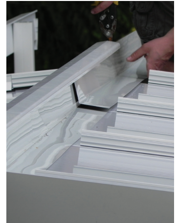
Figure 12. Once the panels are installed, their top edges are covered with lengths of aluminum flashing that tuck up into a downward-facing leg on the ridge beam.
