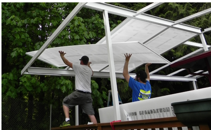
Figure 10. Acrylic roof panels are light, but should be handled by a couple of workers to prevent damage.
