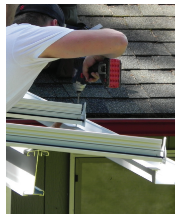
Figure 8. Gutters are included in the patio-cover kit and are screwed to the lower end of the T-bars. Here you can also see the T-bar end caps, which help hold the glazing panels in place.
