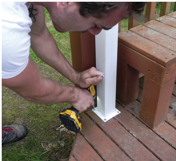
Figure 1. Post base plates are screwed to the bottom of each column and to the deck, which must be properly blocked to support the loads.
