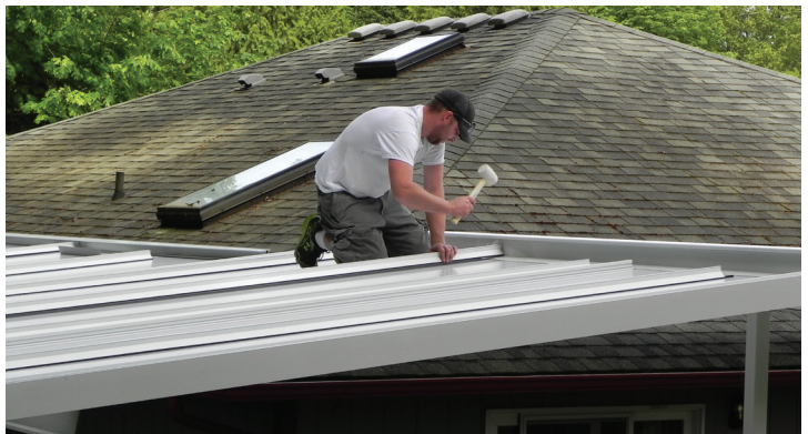
Figure 13. Finally, gasketed T-bar caps are carefully hammered into place over the tops of the T-bars using a rubber mallet.
