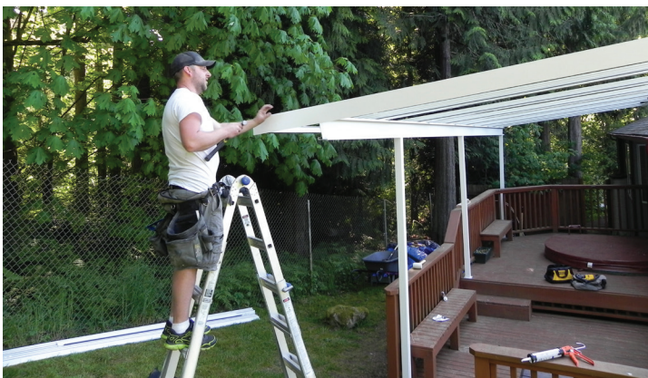
Figure 9. The outermost T-bars are fitted with side fascia trim.
