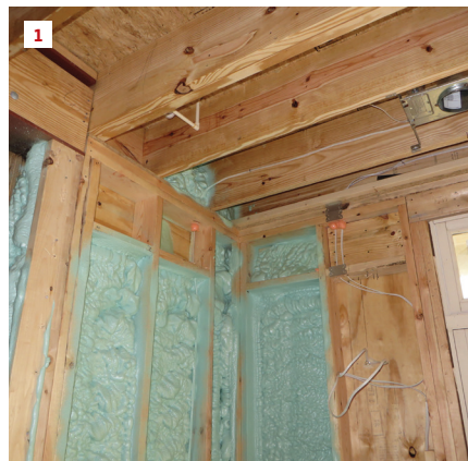
1. Visually, the foam in this wall looks pretty good. 2. On the camera, a flaw in the narrow corner stud bay is clearly visible as a cold (dark) spot.
