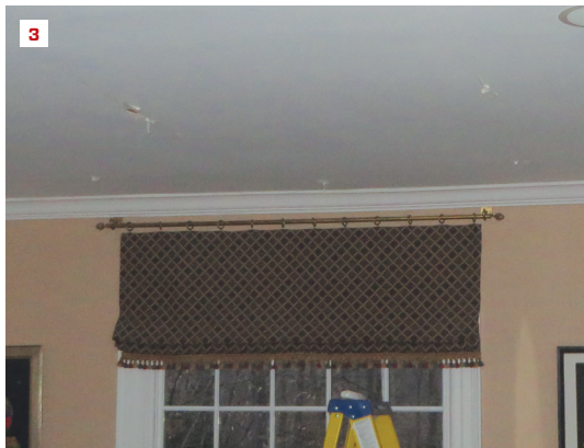
3. We knew some of this ceiling was wet from a bath leak above. But where exactly were the wet areas? 4. With the infrared camera, we could see the wet areas as cold spots (darker colors), showing the extent of the leak.
