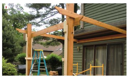
When the beams were level and the posts plumb, I fastened them together with <sup>1</sup>/2-inch-diameter galvanized carriage bolts, removed the braces, and installed
