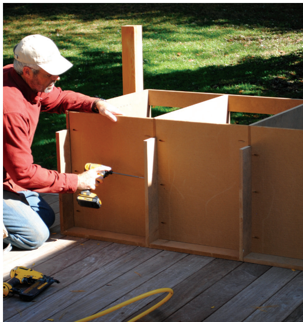
Figure 5. Cabinet bottoms were nailed in place, then more securely fastened with pocket screws.
