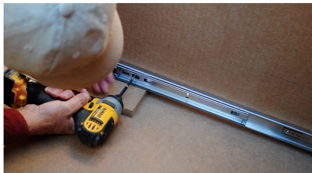
Figure 8. While the drawer slides were being mounted to the cabinet box, temporary 1/2-inch-thick shims were used to hold them off the box bottom.
