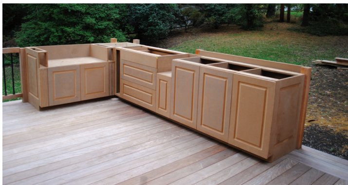
Figure 12. Made from Extira, the outdoor cabinets are ready for painting—inside and out—and for the installation of stone countertops.
