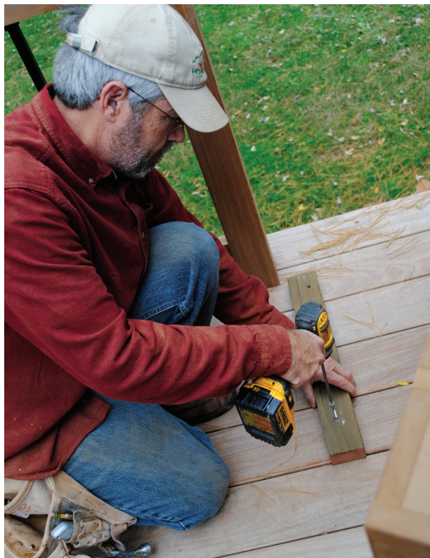
Figure 7. To secure the cabinets in place, the author first screwed cleats to the decking, then screwed through the cabinet side pieces and into the cleats. The cabinet boxes were also screwed to the deck posts.
