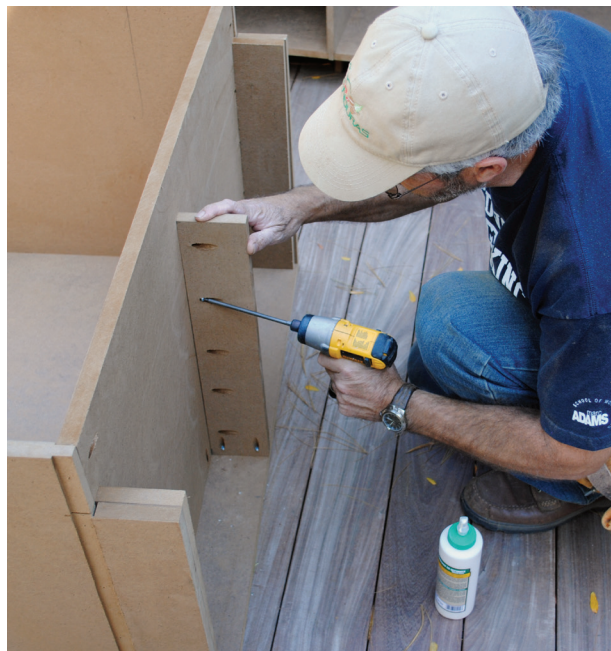
Figure 6. An additional, intermediate support in the toe space and cleats glued and screwed to each side piece reinforce the cabinet that will hold the heavy grill.
