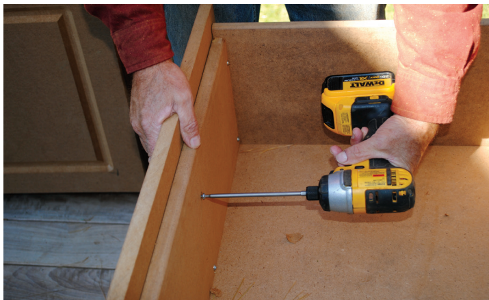
Figure 10. When the drawer fronts were in place, screws were used to attach them from the back.
