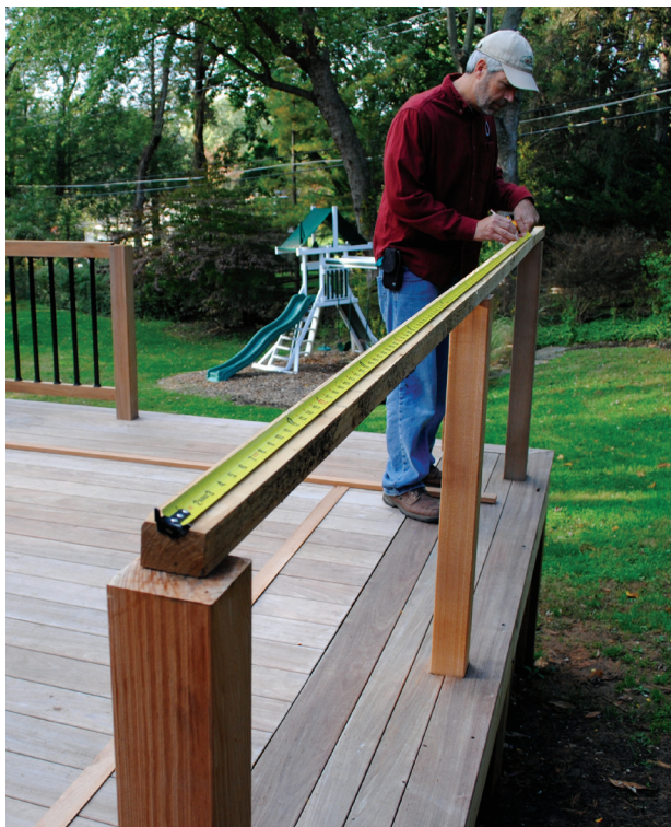
Figure 1. After laying temporary strips on the deck to indicate cabinet locations, the author made a story stick to lay out appliance locations and cabinet partitions.
