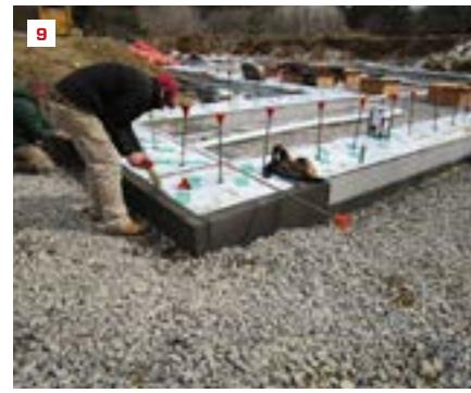
too cold. And in this case, I can tell you that if you were to pull out that footing insulation, that edge of that slab would be cold."
