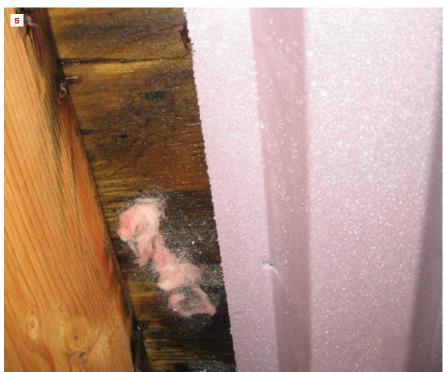
The Kraft facing on the insulation looked fine, but when I pulled the insulation out of a couple of rafter bays, I found saturated fiberglass (3) and saturated plywood roof sheathing (4). In some bays, there was actually frost on the sheathing and insulation (5).
