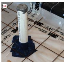
system, preventing any moisture from rising through the assembly and making the slab damp. Another reason for using the polyethylene sheet on top of the rigid insulation was to keep the wet concrete from seeping between—and under—the insulation panels during the installation. We had heard horror stories and seen scary pictures of wet concrete getting under insulation and causing the panels to "iceberg" or float up through the wet mix before it hardened.
