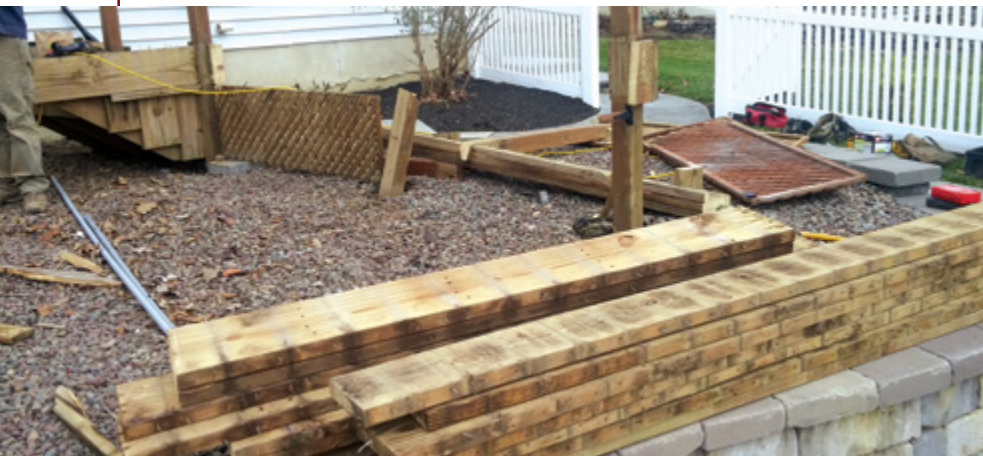
Figure 7. During demolition, old PT framing that is in reasonable shape and that can be reused or recycled is stacked and set aside, rather than sent to the landfill.
