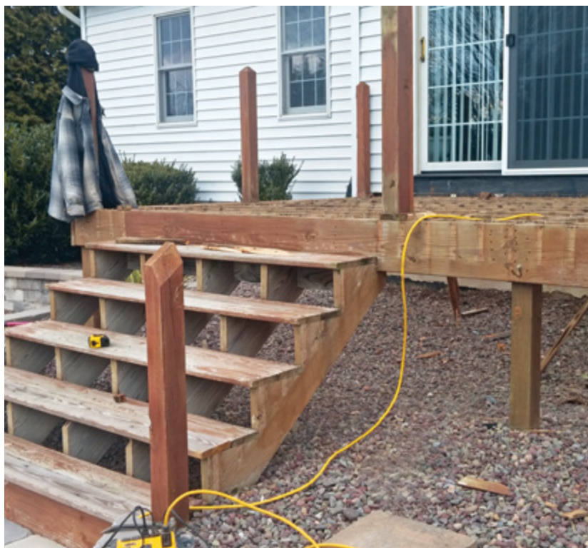
Figure 3. A typical demolition job starts with rail removal, followed by the decking. For easier access, the steps are left in place until it's time to remove the framing.
