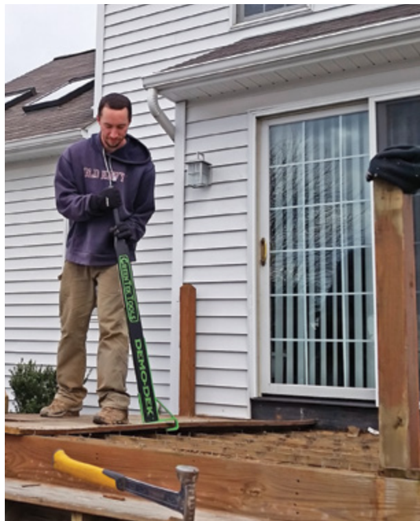
Figure 2. The author's crew also uses the Demo-Dek ( greentektools.com ). It has a jaw design that doesn't require a joist or beam for leverage, and that holds the deck board in place after it has been removed.
