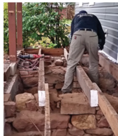
Figure 3. A typical demolition job starts with rail removal, followed by the decking. For easier access, the steps are left in place until it's time to remove the framing.
