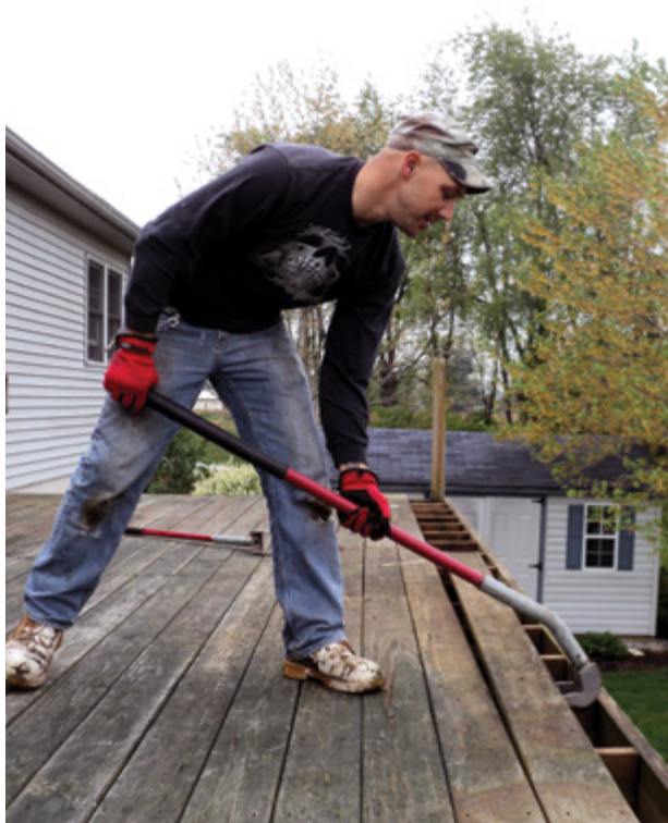
Figure 1. The author's crew uses several different decking-removal tools, including the Duckbill Deck Wrecker ( deckwrecker.com ), which has steel jaws designed to straddle single or double 2-by framing.
