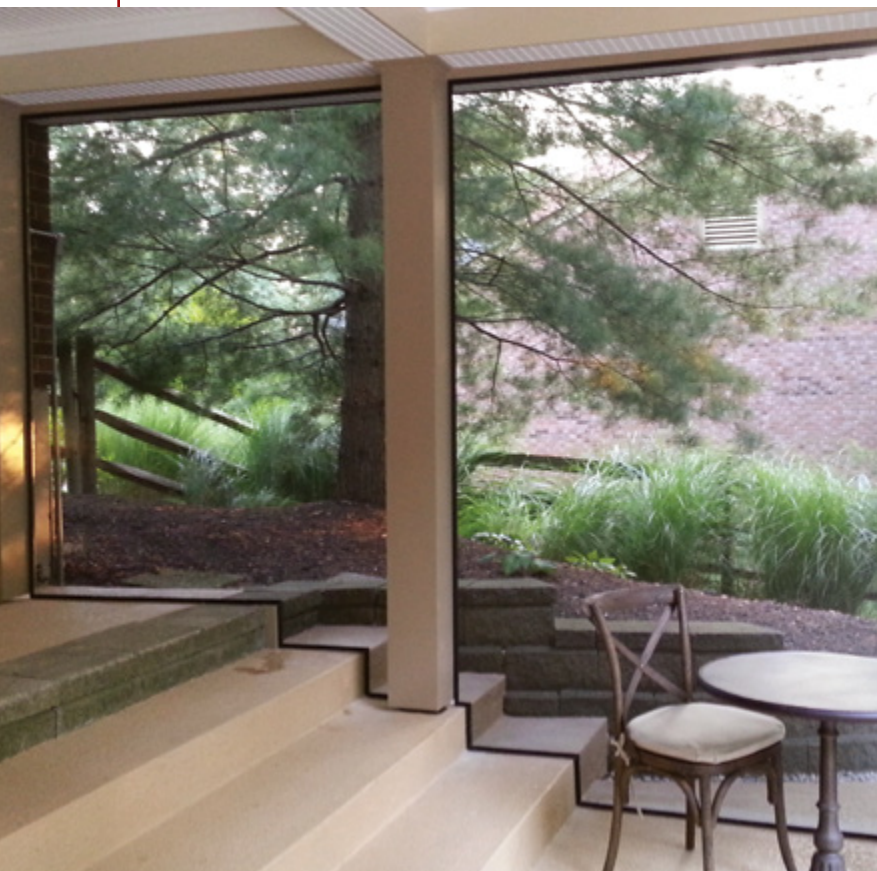
Figure 2. Instead of relying on rubber splines, ScreenEze has a vinyl cap that snaps over its \frac{3}{4} -inch by \frac{3}{4} -inch aluminum base channel (above). The system has a minimal, unobtrusive profile that fits well with contemporary designs, and can span openings up to 150 square feet (left).
