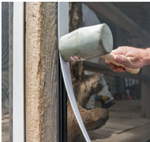
Figure 1. While most screen track is made of extruded aluminum, Screen Tight also offers a UV-protected vinyl profile (top). After the screen has been attached to the base with splines, a removable vinyl cap is snapped onto the base, which evenly tightens the screening (above).
