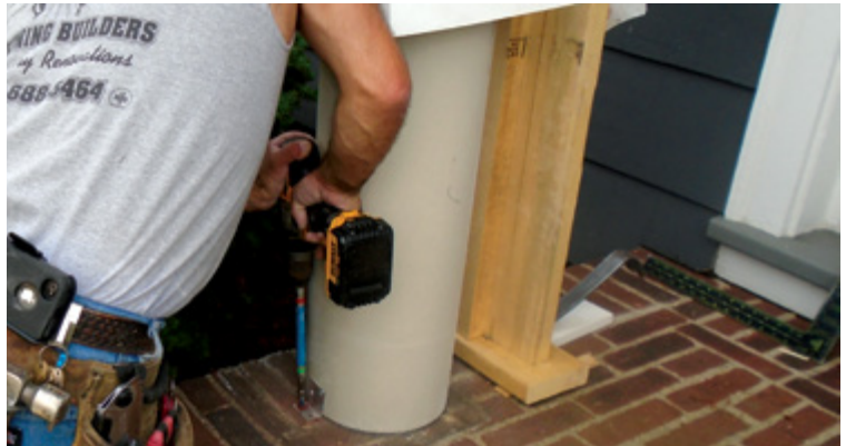
Figure 6. The bases of the columns were secured to the porch with \frac{5}{16} -inch-diameter by 2\frac{3}{8} -inch-long Tapcon masonry screws driven through the installation clips and into holes drilled into the brickwork.
