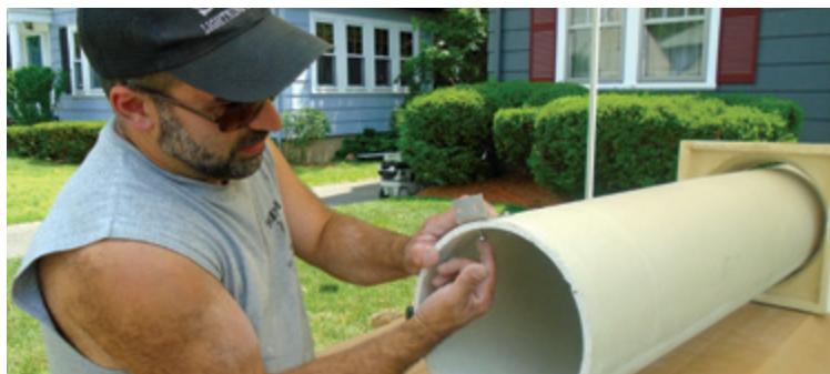
Figure 4. The author used stainless steel bolts and nuts instead of the supplied screws to fasten the installation clips to the column bases.
