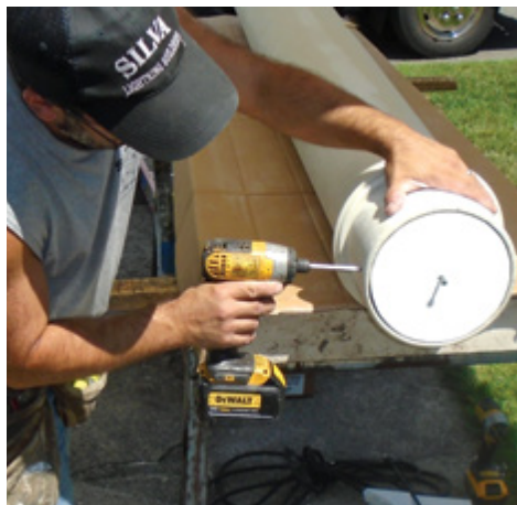
Figure 2. The author extended the columns by first inserting a plug made from a double layer of \frac{3}{4} -inch-thick PVC into the top of each column (above left). The plug serves as an attachment point for another, slightly larger PVC plug that's sized to match the outside diameter of the column and routed with a channel to fit into the flashing cap (above right). The column extensions effectively lower the position of the column's decorative trim rings.
