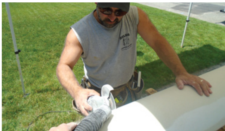
Figure 3. A 4½-inch angle grinder equipped with a diamond masonry blade was used to cut the columns to length.
