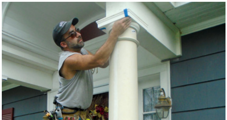
Figure 7. After gluing the capitals to the flashing caps with OSI Quad Max sealant, the author used masking tape to hold the capitals in place until the sealant cured.
