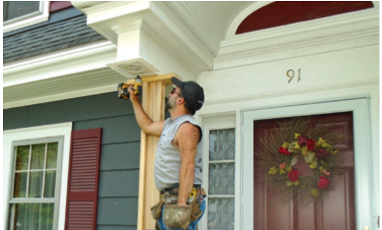
Figure 5. The top of the column fit into a flashing cap that was screwed to the underside of the beam.
