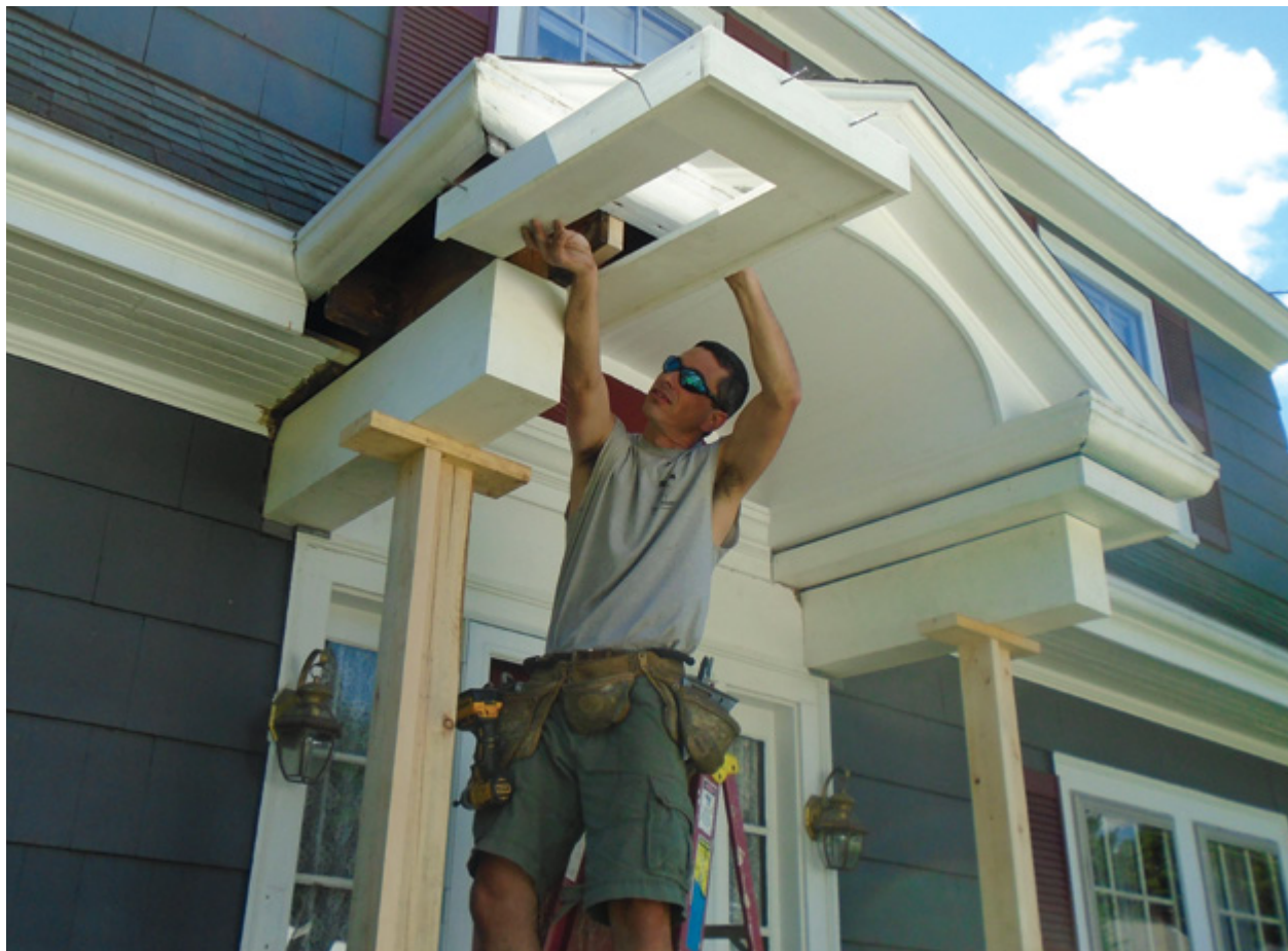
Figure 1. The original beams—which were actually framed like short knee walls and clad with board sheathing—had water damage, so the author reframed them with PT lumber and clad the new beams with PVC trim. Then he prefabricated U-shaped PVC soffit/fascia assemblies and slipped them into place.
