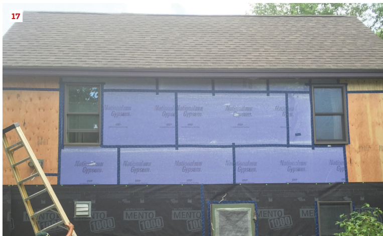
After resheathing the newly insulated walls with vapor-open Gold Bond gypsum board (15) and taping the seams with Tescon Vana tape (16), the crew covered the sheathing with Solitex Mento 1000 (17).
