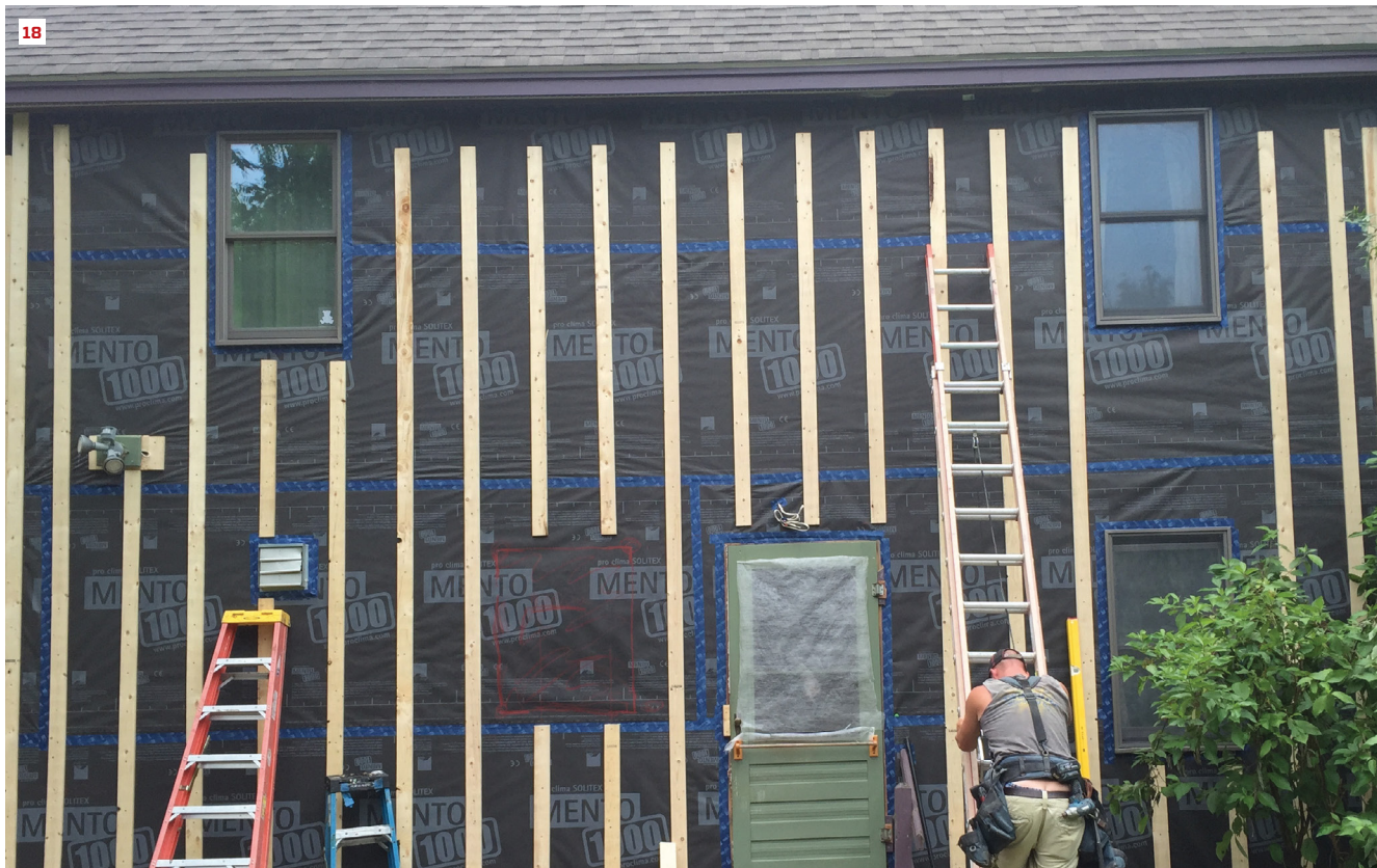
Over the vapor-open Solitex Mento 1000 weather-resistive barrier, the crew applied 1x4 strapping to create an air channel behind the new fiber-cement lap siding (18).
