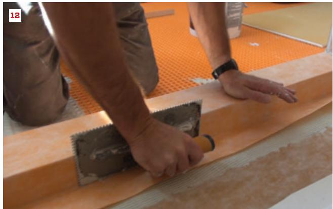
The author cuts two pieces of 2-inch-thick Kerdi-Board to length (9) before bonding them together with unmodified mortar to make his shower curb. He applies a measured amount of modified mortar to the subfloor (10), combing it out with a 1/4-inch notched trowel. After pressing the curb into the mortar and allowing the bond to cure overnight, he applies unmodified mortar to the curb using a Kerdi trowel with 1/8-inch notches (11), then presses Kerdi membrane into the curb (12).
