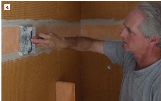
The author cuts 1/2-inch-thick pieces of Kerdi-Board to size using a utility knife (1), then fastens the board to the shower wall framing using screws and special toothed washers (2). He applies unmodified mortar to the joints using the 1/8-inch notched Kerdi trowel (3), then presses Kerdi-Band membrane into the mortar to waterproof the joints (4). He will also apply mortar and Kerdi-Band to the washers and screws used to attach the Kerdi-Board in the field.
