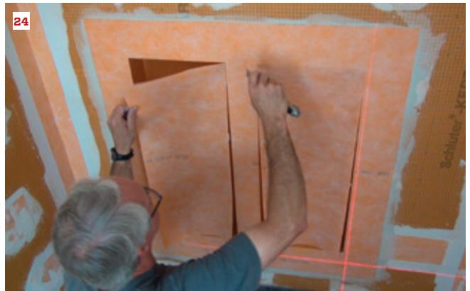
Guided by a laser level, the author traces the outline of a preformed recessed shelf box on the already waterproofed wall (21), then cuts out a section of Kerdi-Board and removes it (22). After setting two boxes into two adjacent stud cavities, he fastens the boxes in place with screws and washers (23). He applies mortar over the joints between the boxes and the wall, then presses a large sheet of Kerdi membrane into the mortar before cutting out the box openings with a knife (24).
