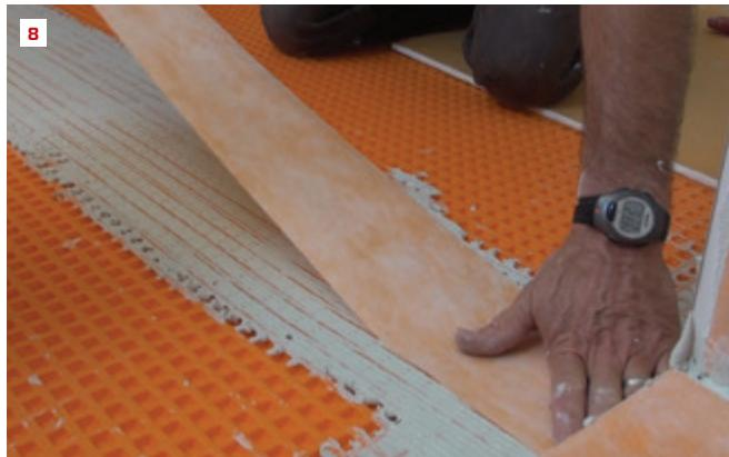
The author cuts Ditra floor membrane with a utility knife (5); combs out a measured amount of mortar using a trowel with 1/4-inch notches (6); lays a sheet of Ditra into the fresh mortar (7); and applies a strip of Kerdi membrane to the joint between two sheets (8). Modified mortar prepared using an acrylic latex admixture bonds the Ditra to the Advantech subfloor, but unmodified mortar is used to adhere the strips of Kerdi membrane to the Ditra.
