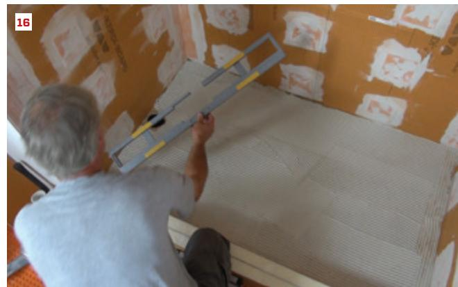
The author attaches a PVC pipe fitting to the Kerdi-Drain linear drain using a FernCo coupling (13), then test-fits the drain to the pipe stubbed up under the floor (14). Next he applies modified mortar to the Advantech subflooring (15) and sets a polyethylene foam support into the fresh mortar (16). This piece will supply firm support to the linear drain and bring the drain flush with the sloped Kerdi-Board shower floor pan.
