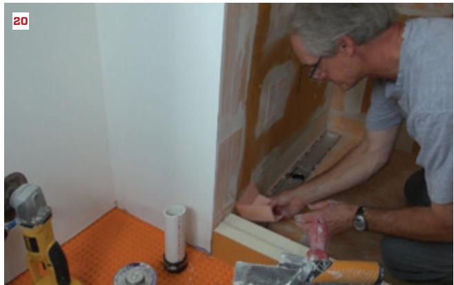
The author sets the tapered Kerdi-Board shower pan into the freshly applied latex-modified mortar (17), then trims the corners of the linear drain's pre-applied Kerdi membrane (18). He trowels unmodified mortar onto the waterproof facing of the pan (19). After applying PVC cement to the linear drain's collar and setting the drain in place, he presses the drain's pre-applied membrane into the fresh mortar, then covers the cut corners with preformed Kerdi corner pieces (20).
