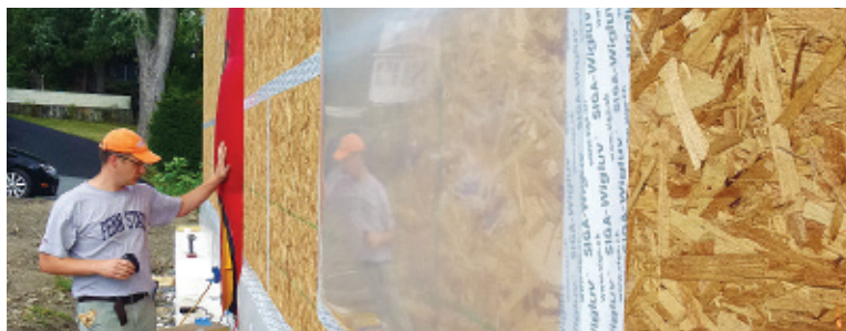
Architect Richard Pedranti, HERS rater Pete Vargo, consultant Bryan Kehm, and builder Rob Ciervo tape plastic over the OSB sheathing during a blower-door test (top). At bottom, the plastic balloons out under air pressure.
