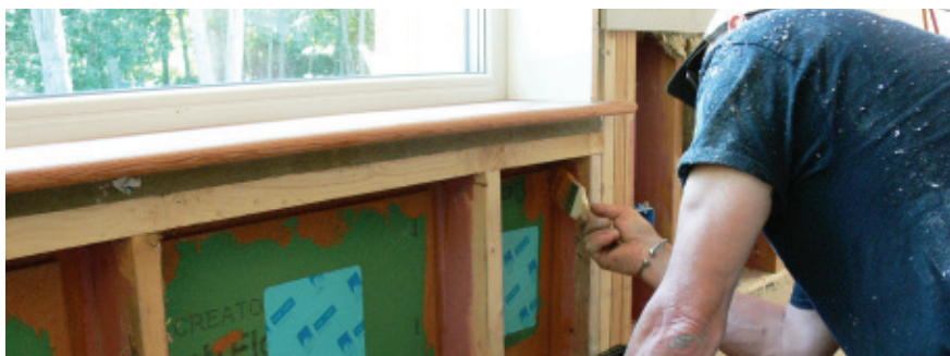
After a plumbing break flooded a newly built Passive House, an EcoCor crew cut open the OSB air barrier to remove damp insulation from the outer cavity (top), then patched the holes (bottom) with Zip sheathing, Pro Clima Uni Tape, and Prosoco R-Guard Cat5.
