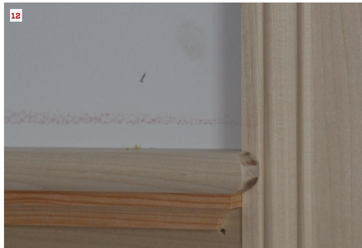
the casing started with a flat return about  $\frac{1}{2}$  inch wide. I made the return on the cap so that it ended on the flat part of the casing just before the rest of the profile began. Then I routed a bullnose on the return with a  $\frac{1}{2}$ -inch round-over bit.
