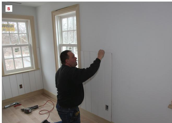
A lot of carpenters would start running the sheets at one corner and work their way across the wall. But with the layout set, I actually started by installing the piece that went around the outlet and one corner of a window. That piece would key in the placement of the rest of the pieces on the wall.
