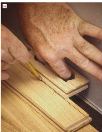
needs to be cut. I mark three or four courses and then square the mark across each board (25). Next I put the boards together with the cut lines lined up. I set the saw track in place and cut the ends, again at a slight back bevel (26). As I set each board into place, I try for a snug fit without forcing the board. If the fit is too tight, I finetune it with a rasp so that the board goes in without pushing the baseboard over.
