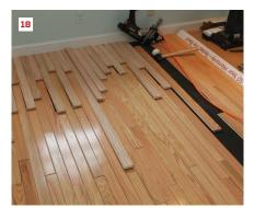
so I remove them. I also remove the string, but I keep the nails in place so that I can check the straightness of the first course after it's installed.
