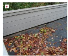
flashing can create a dam that holds water (2). If you're the one sloping the roof, adding pitch here can help the water run off, but we often need to work with what's already there.
