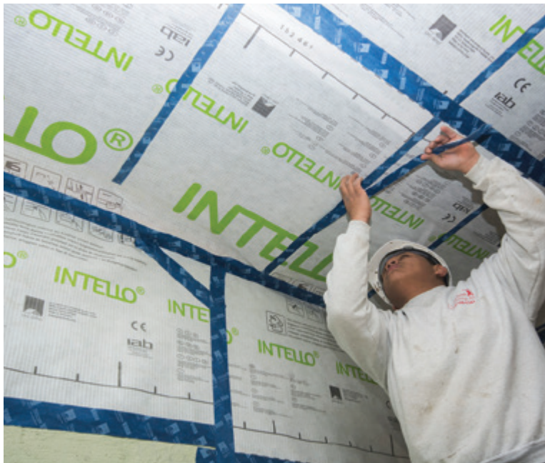
A technician for J's Custom Contracting installs Intello smart vapor barrier on the ceiling under the low-slope roof of a Brooklyn, N.Y., row house. Flat roofs, which are tricky to vent, are one case where smart membranes can be problem solvers.
