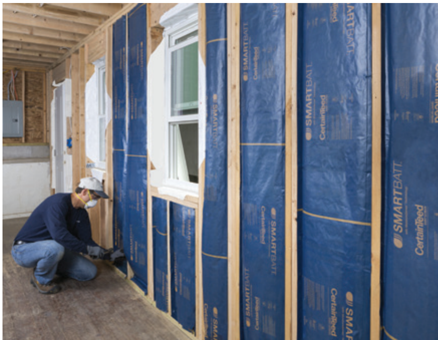
A worker installs CertainTeed SmartBatt fiberglass batts into a stud cavity in this photo supplied by CertainTeed. Applied in this manner, the product helps manage vapor diffusion, but will not serve as an air control layer.
